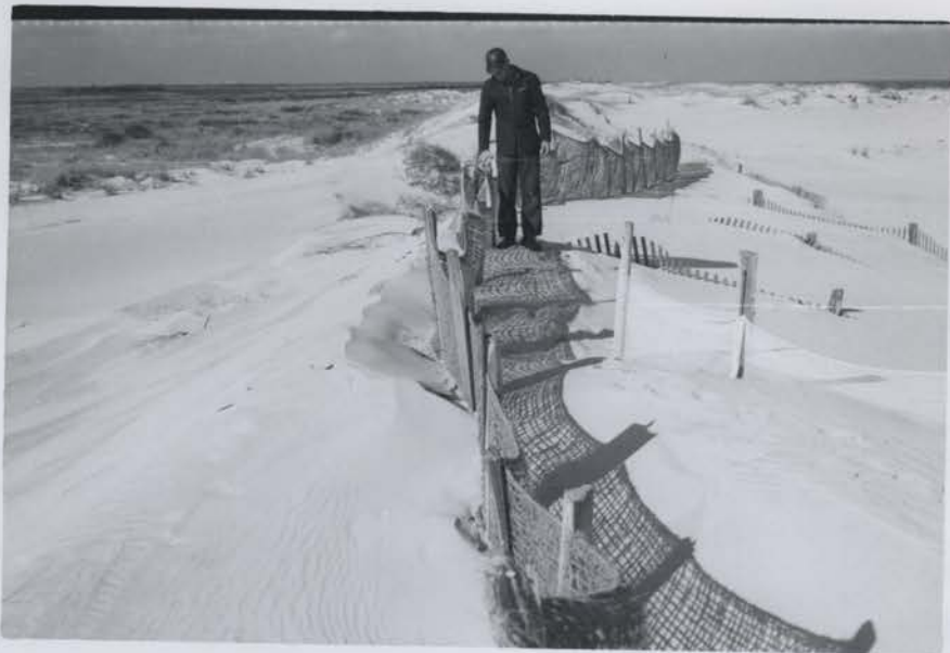
Experimental sand fence panel of Ludlow Heavy Duty Soil Saver. Erected November 19, 1959; photo taken December 29, 1959. Material is jute, 45" wide; 150' / roll; weight/roll 90#; cost per roll for 3 or more rolls $13.65. Same length of snow fence would weigh 390 lbs. and cost $28.50. Also available in regular duty weight, which is of closer weave and, I believe, better adapted for this type of thing. Regular material is 50" wide, 225 ft./roll; 90#/roll; $15.60/roll for 3 or more rolls. Sand was blown from viewer's right with NE wind. Note that sand is piled on both sides of panel. Pine slabs spaced 6'. Material secured to slabs with thin strips of wood. Note that material passes on alternate sides of pine slabs; this provides more strength. R-19-6, December 29, 1959.
