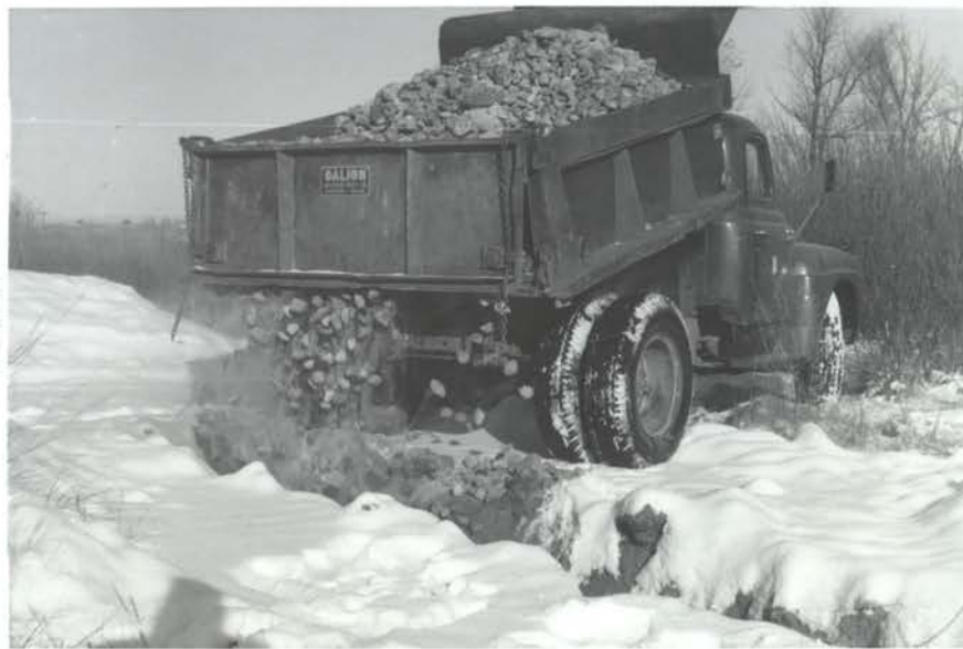
Dumping gravel into lateral drainfield addition. Roll 133 Exp.8
