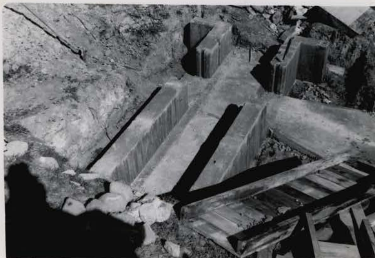
R-86, E-5 (4/16/54) Bowdoin. Three-way irrigation turnout structure at outlet to headquarters irrigation reservoir.
