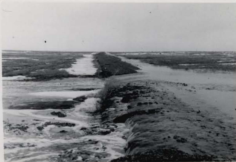
R-86, E-4 (4/6/54) Bowdoin. Runoff from melting snow going over patrol road south of G.N. tracks. This flow caused mainly by break in south Reclamation canal that picks up runoff from hills to the south of refuge.
