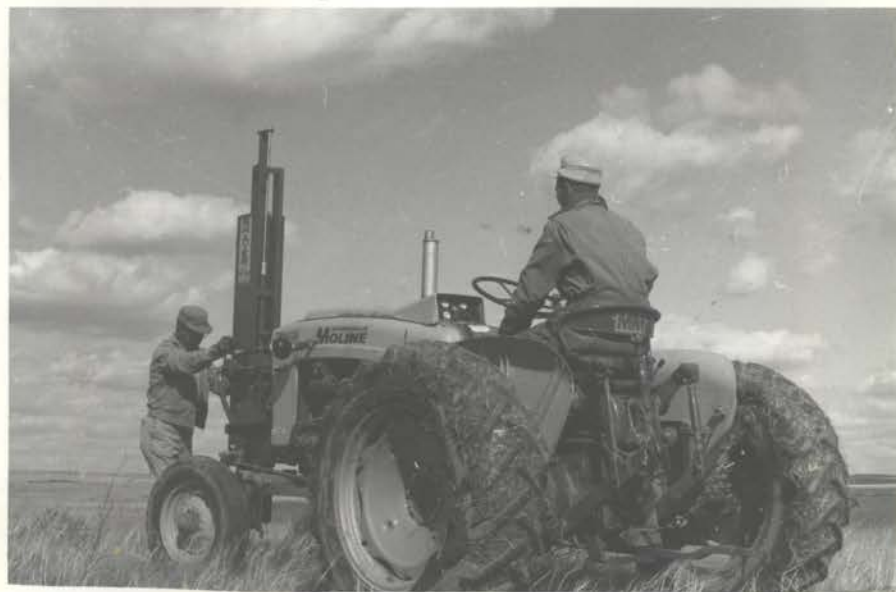
Our new "Shaver" post driver was happily received and works wonders building fence. Many man-hours saved by it. Roll 150, Ex. 10.
