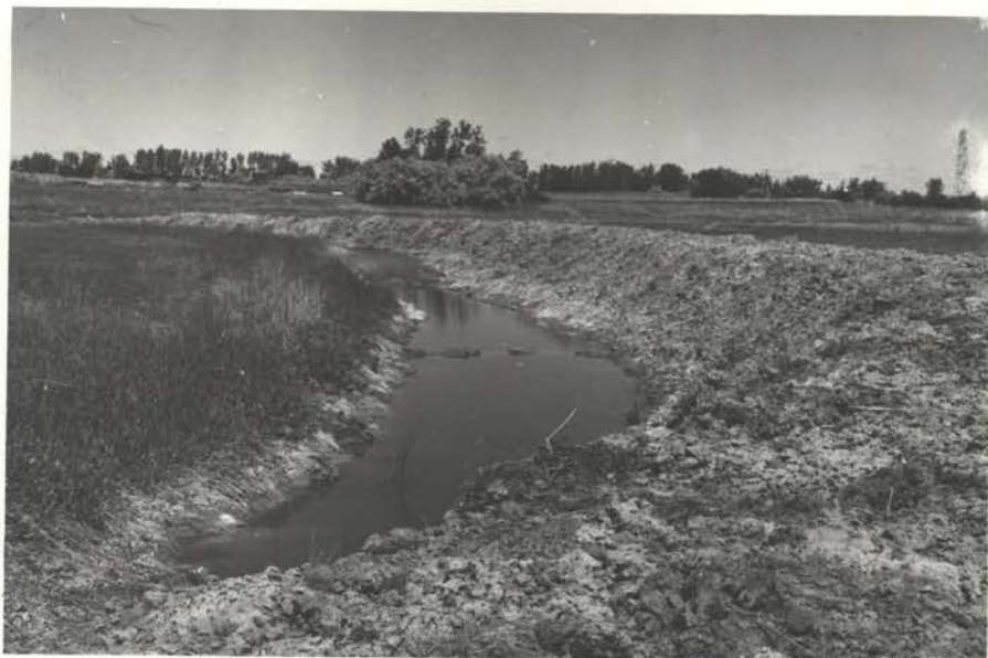
Dike #1 Black Creek Coulee construction to hold back wasted seepage and runoff water. Roll 146, Ex. 8
