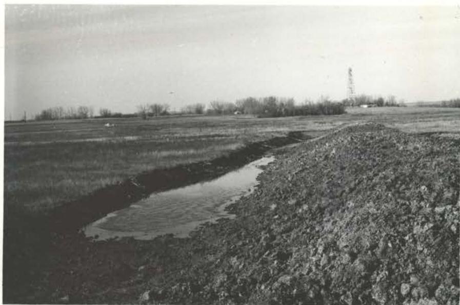
The beginning of Dike #2 accomplished with a dragline. Looking northwest. Roll 151, Ex. 18
