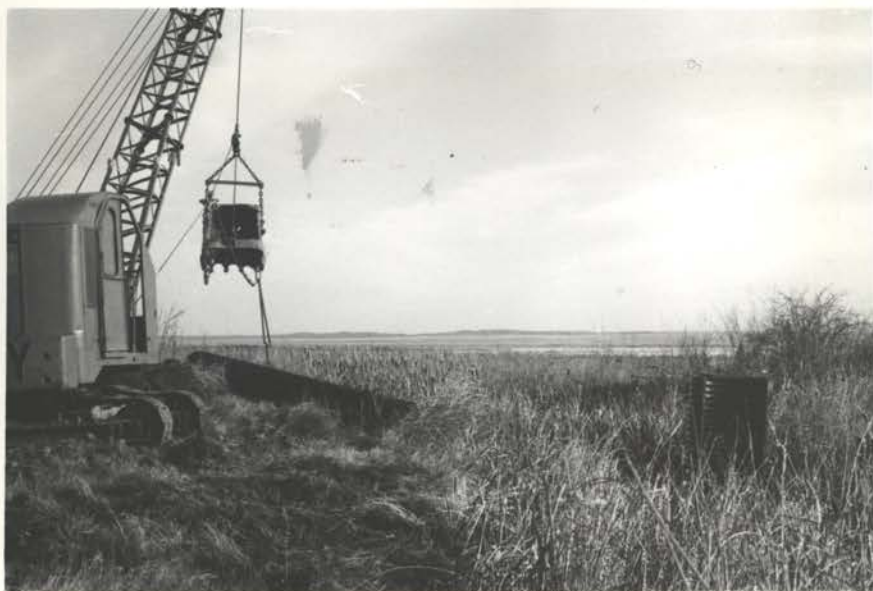
Putting the water structure in Dike #2, a S&M project, Roll 151, Ex. 4
