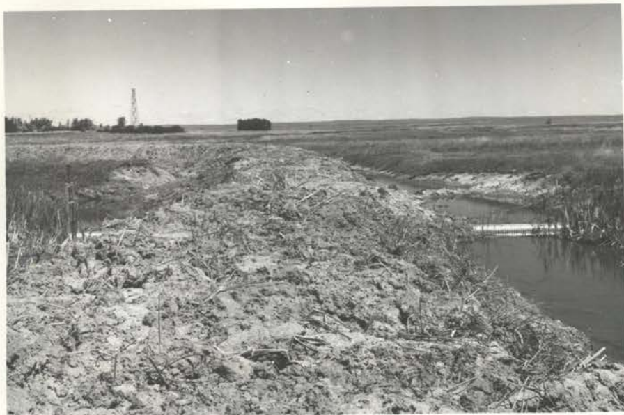
Dike #1 Black Creek Coulee ponding construction project showing drainage culvert in place. Roll 146, Ex. 3
