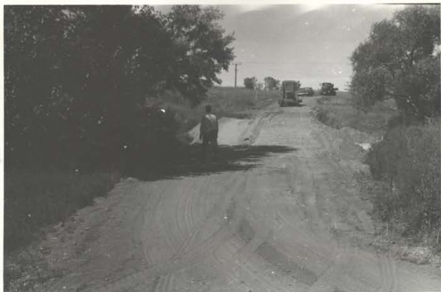
Black Creek Coulee crossing at SW side of refuge. The culvert was lengthened and repaired. A rock crossing built to take care of flood waters. Roll 147, Ex. 3
