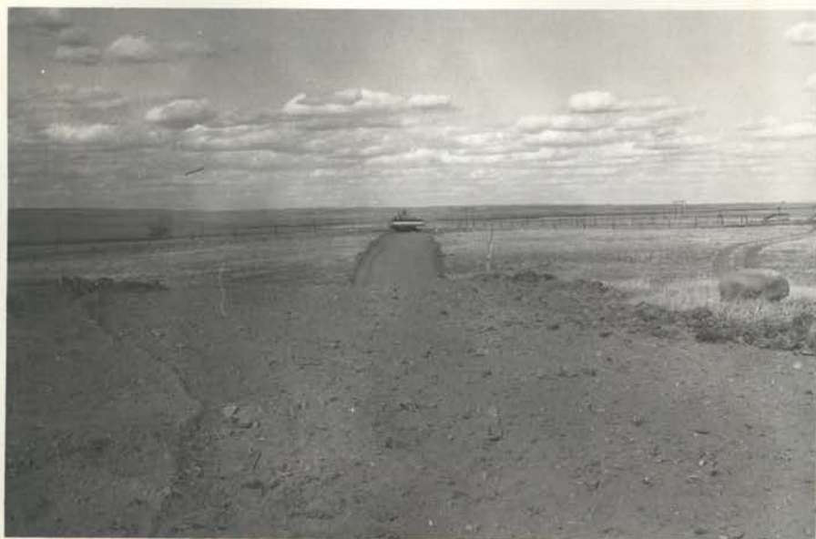
A badly needed road was built connecting the two roads past a branch to control traffic to eliminate scattered trails from getting started. This is also used as a road to a new view point overlooking Bowdoin Lake. This will be surfaced with gravel. Looking NE. Roll 149, Ex. 11
