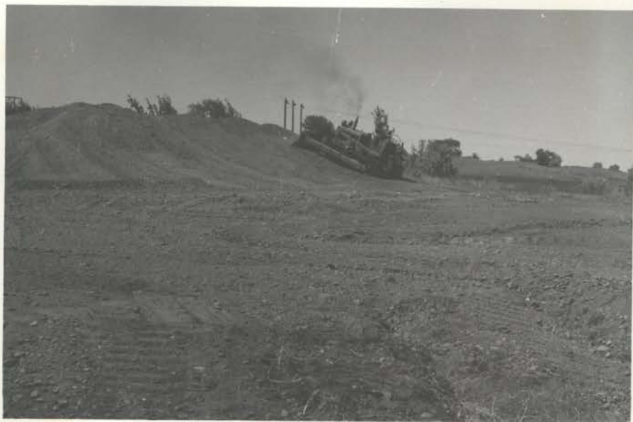
Taking down a steep hill on the patrol trail eliminating a traffic hazard and providing a small mountain of precious and needed gravel. Roll 147, Ex. 12
