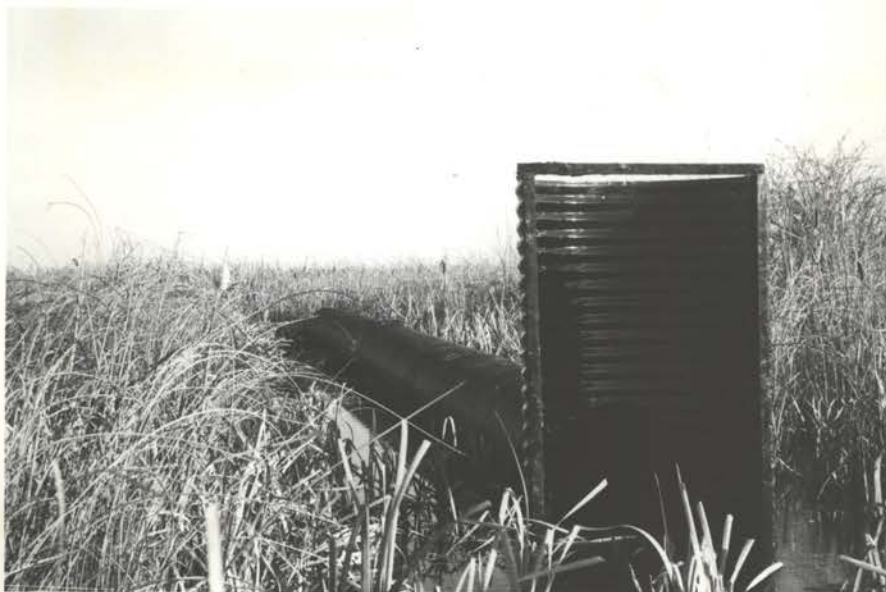
The flash board riser water structure to be used in Dike #2, a S&M project. Roll 151, Ex. 9
