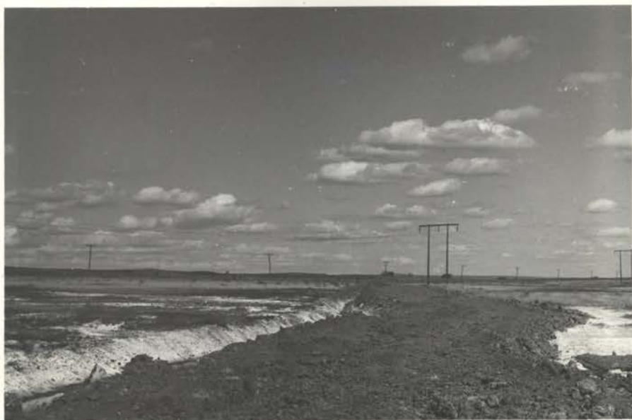
Ditch spoil leveled and seeded. Photo taken northeasterly. Roll 149, Ex. 8
