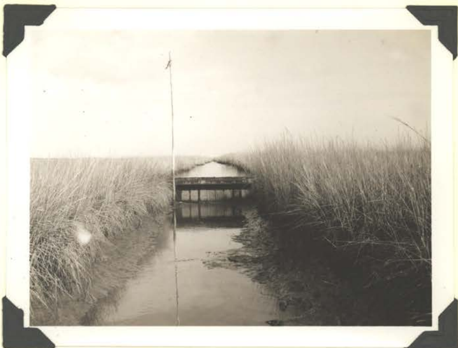
Picture shows plugged mosquito ditch about 2 hours before low tide. Located south of Great Creek Road. 11/11/40
