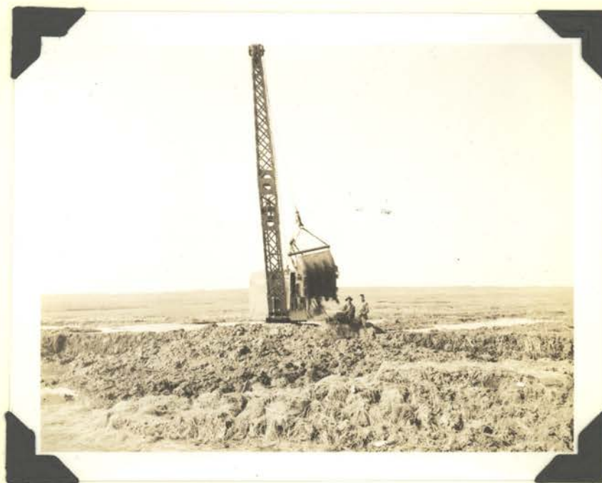
Drag line in operation on dike north of Great Creek Road. 9/16/40
