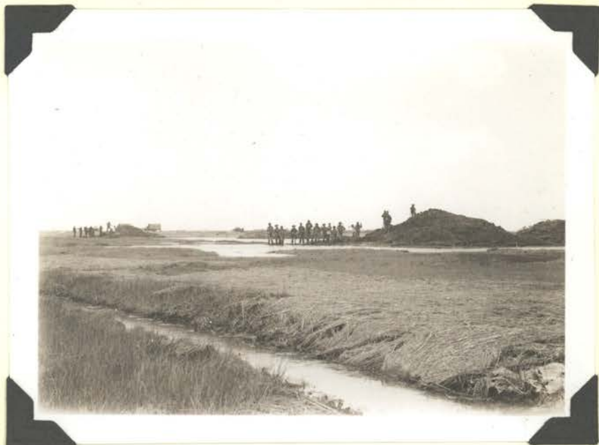
CCC enrollees constructing salt pond and nesting island on marsh between WPA Road and Reed Bay. 5/28/40
