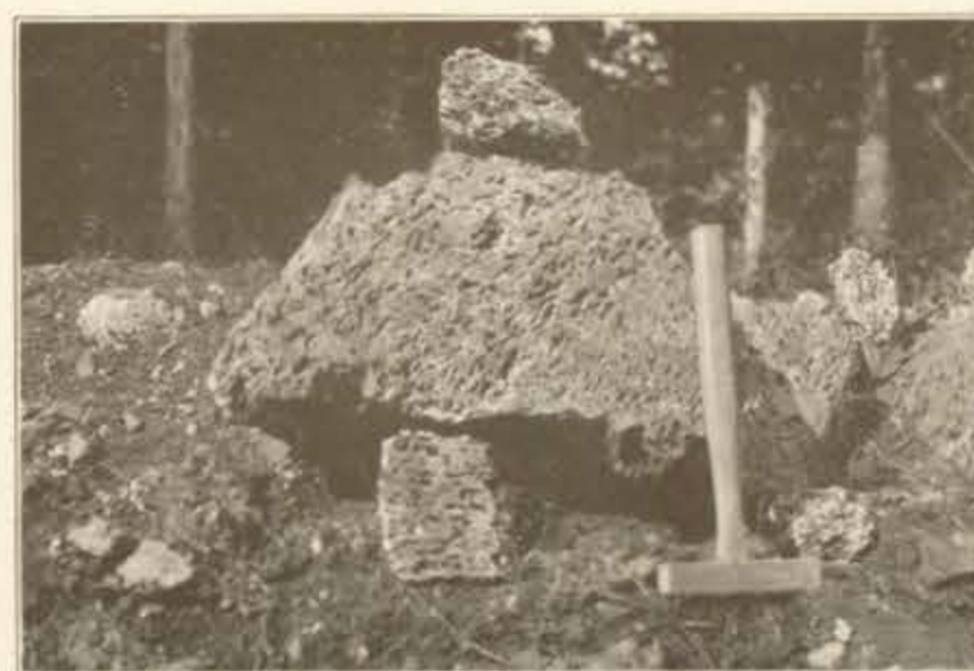
PLATE VI.—CAVERNOUS FOSSILIFEROUS CHERT CHARACTERISTIC OF CHEPULTEPEC DOLOMITE, FROM EAST BASE OF NEWHOPE RIDGE IN GORGE OF BUCK CREEK BETWEEN HELENA AND PELHAM
