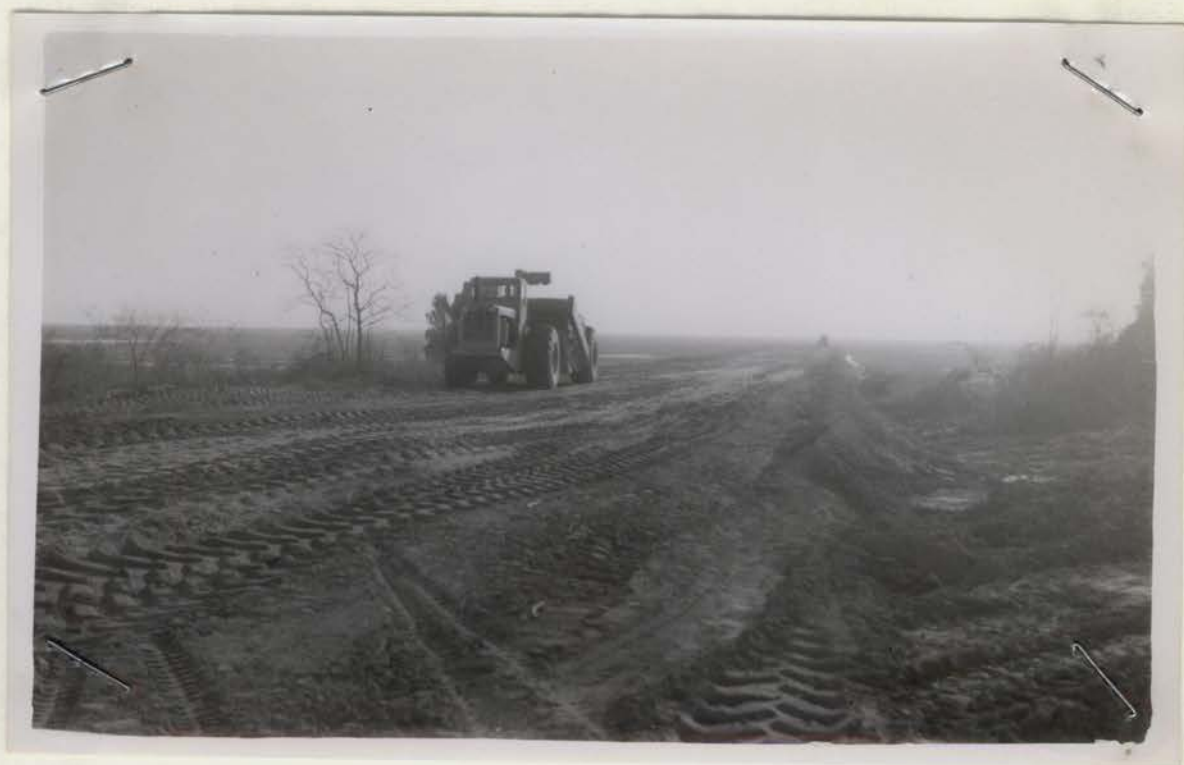
Contractor's Tournapull at Station 2 on way to be loaded
