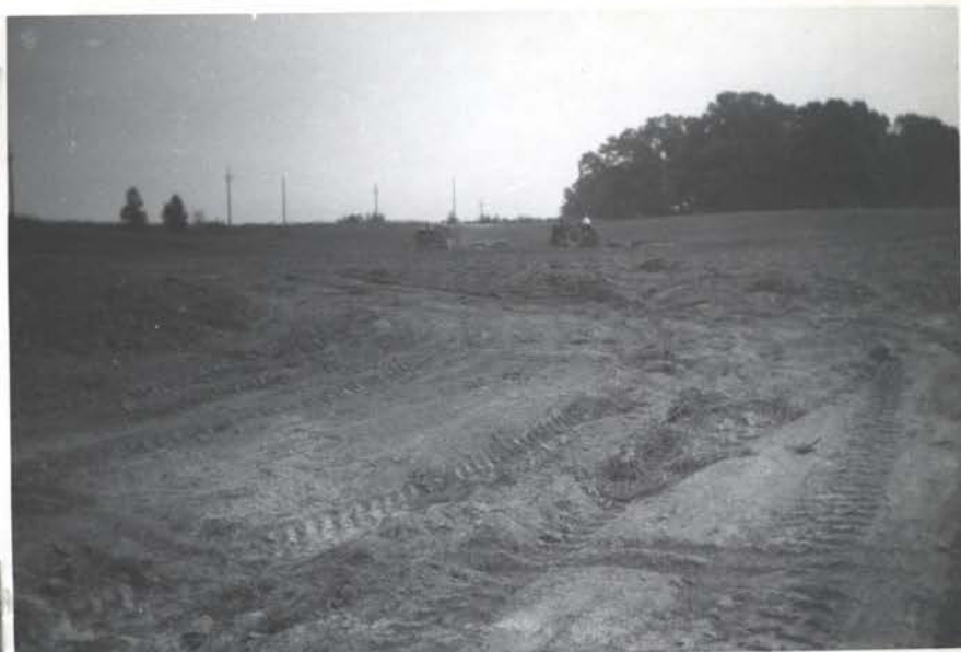
No. 9 - Gully erosion (grader tracks curving to left from foreground represent leveling of a 2 to 4 foot ditch) followed by grass & grain seeding operation. 9/28/50 - G.L.W.
