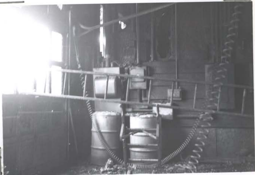
No. 13 - Meter- panel-board; source of our refuge maintenance shop fire. 12/16/50 - E.E.C.
