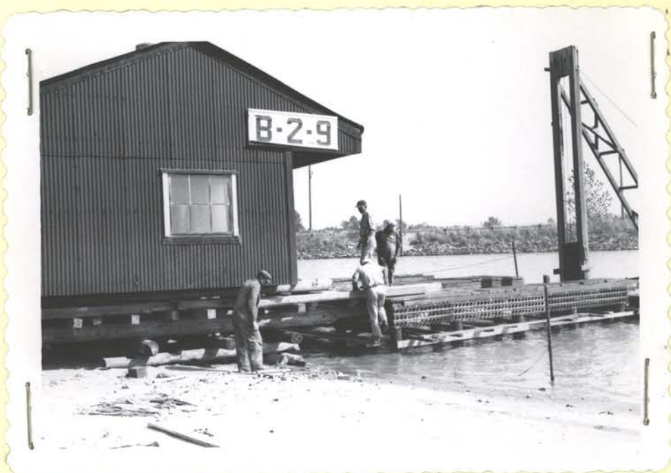
# 3. - Moving of first of two 14' x 24' buildings onto boat-dock deck. 10/1951 - EEC.
