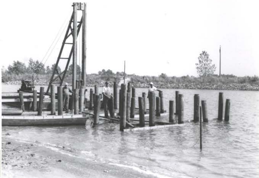
# 1. - Pile driven in place for combination boat-dock boat-house. 10/1951 E.E.C.
