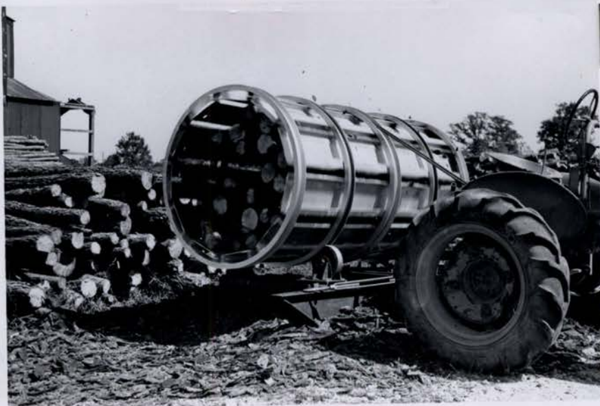
# 5. Refuge made barking machine, patterned after TVA post peeler, in operation barking short-leaf pine posts. Sept. '54 - EEC.
