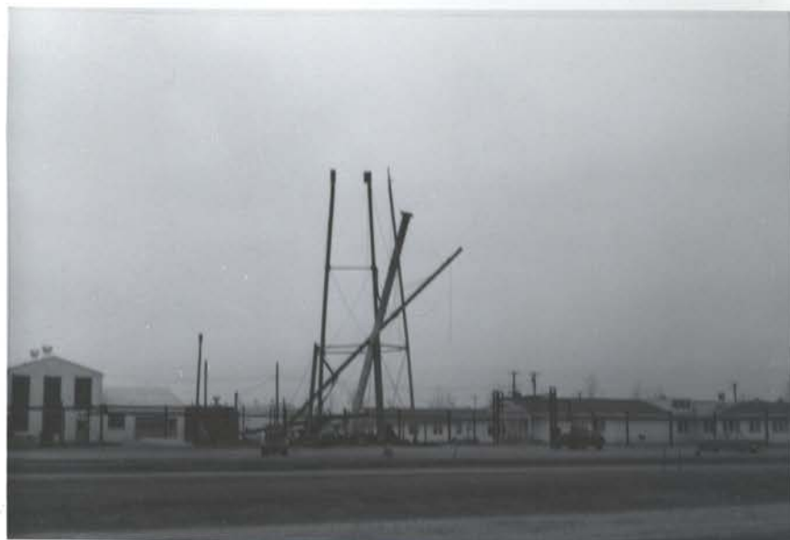
Photo No. 59-5. Tower leg hangs over Vocational Technical Institute Cafeteria like the Sword of Damocles. It took two motor cranes to right structure and lower to ground. January 26, 1959 G.H.H.
