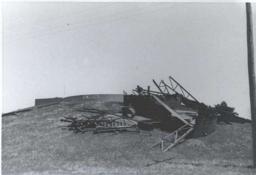
Photo No. 59-9. Scrapping old sewage digester tank cover at Sewage Disposal Plant. Under contract, scrap becomes property of contractor.
