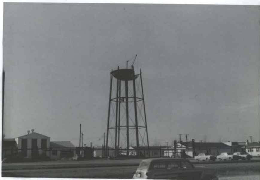
Photo No. 59-4. Trouble! "Fly-by-nite" contractor lost control of leg which fell carrying standpipe with it. January 26, 1959 G.H.H.
