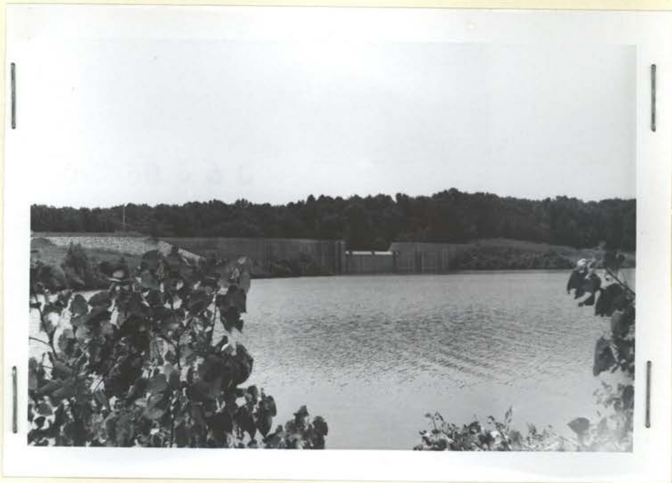
The new Devils Kitchen Lake filled to an elevation 20 feet below spillway. R-6-7 & R-6-8. 6-60, Stiles.
