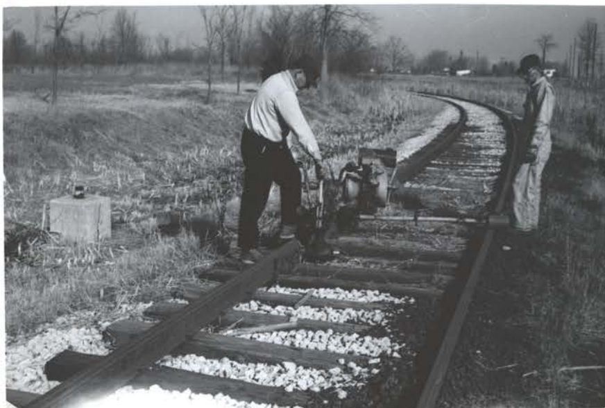
Tightening track bolts with machine on loan from Illinois Central Railroad. Track-bolt tightening on 29 miles of "Crab Orchard and Southern" this period completes three-year rehabilitation of our line. R-1-6 H.S. 2/5/62.
