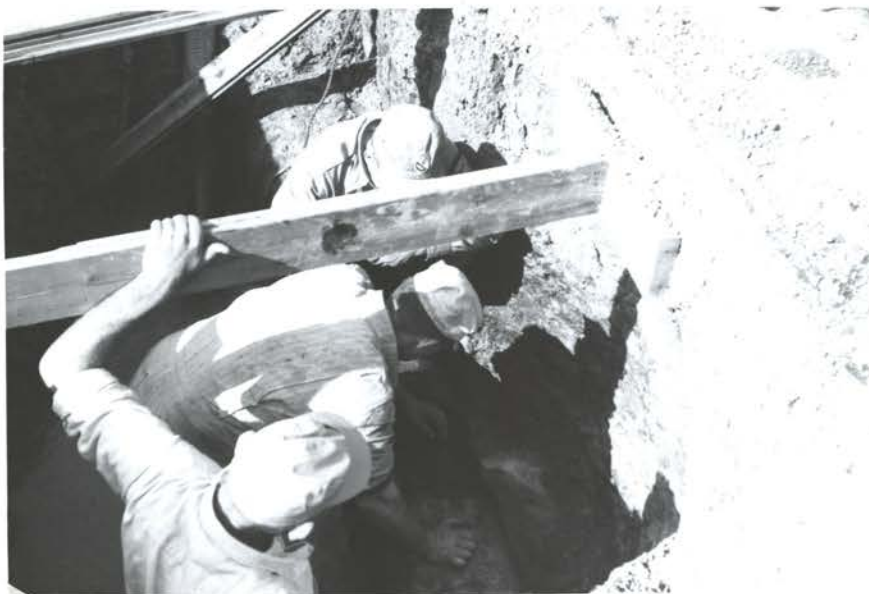
As usual, a hole in the steel Dresser coupling--the weak links in this section of our main water distribution system. R-4-7 C.B. 4/17/62.
