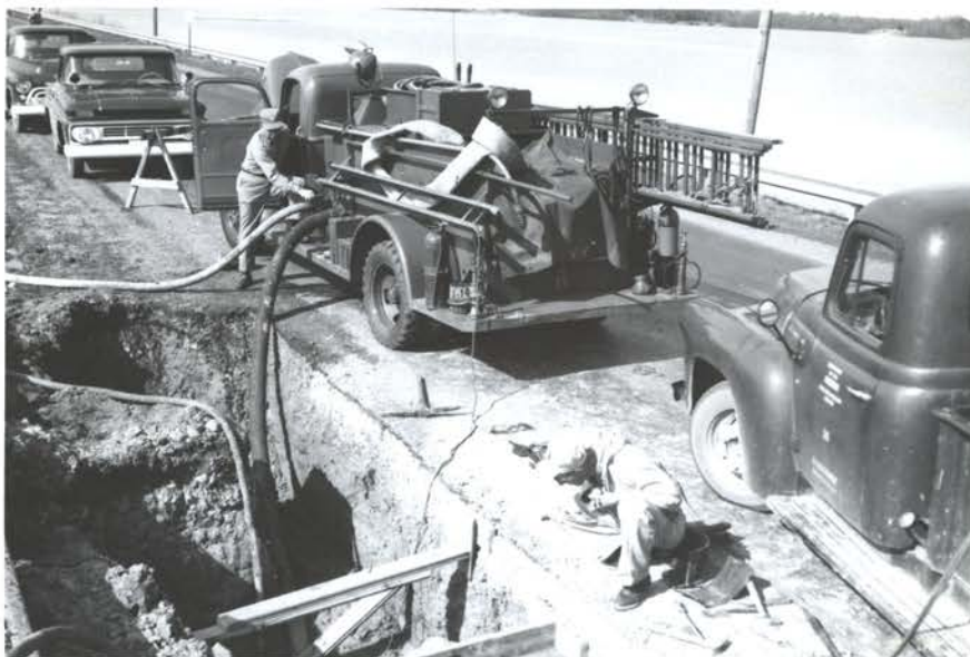
Pumping seepage water from excavation made to repair 16" water main. Capacity of fire pumper needed to hasten repair and get pressure back to normal at refuge industrial tenants on South side of lake. R-4-8 C.B. 4/17/62.
