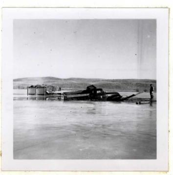
It was impossible to pull the truck back on top of the ice without risking severe damage to the rear end and we therefore employed dynamite to blast a path to the shore. We were fortunate in that the wind was blowing away from the vehicle and therefore the debris did not fall on the truck. We used not more than two dynamite sticks at a time so that the possibility of concussion damage was held to a minimum.
