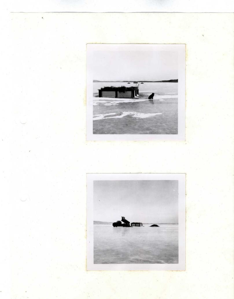
This is the manner in which the islands settled even when they were only partially filled. After such settling started, it was unsafe to use any equipment in the immediate vicinity.
