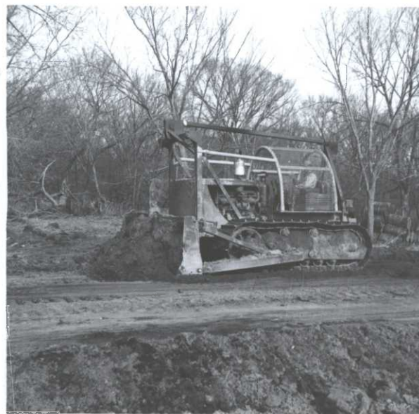
3/28/62. Surplus D-7 acquired from National Guard at Topeka, Kansas. Tractor is in very good condition. Note brush guard installed for material cost of about $105.
