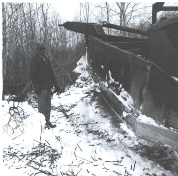
3/7/62. Contractor Bill Lee with his tree cutter mounted on front of D-8. He was hired for 150 hours of work @ $16.50. He cut 120 acres for an average cost of just over $20 per acre.
