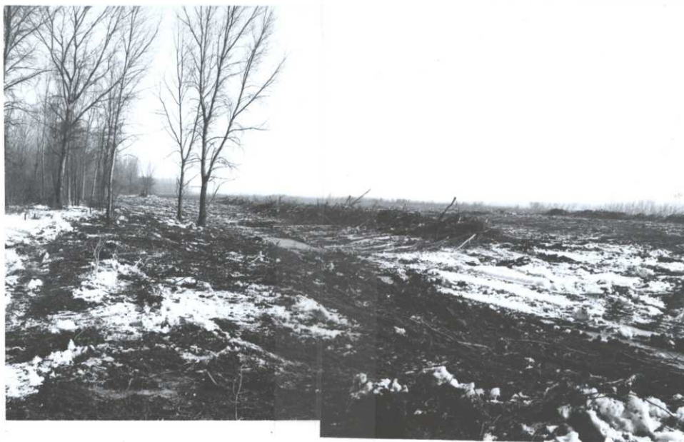
3/15/62. Windrowing brush and trees with refuge D-7. Material was cut off at ground level with a tree cutter. The stumps of cottonwood and willow will rot out in about three years. This area along the east side of the "island" will be used for goose pasture.
