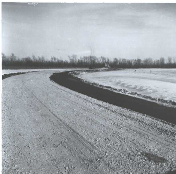
1/13/62. Nearing completion of hauling and spreading 10,000 tons of crushed limestone on loop road.
