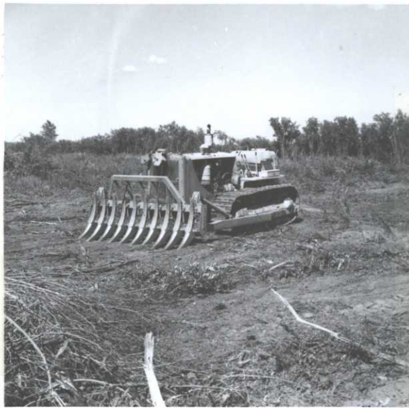
Rental brush rake (Fleco) used in land clearing. Rake is mounted on D-8 received as surplus property from Fort Leonard Wood.
