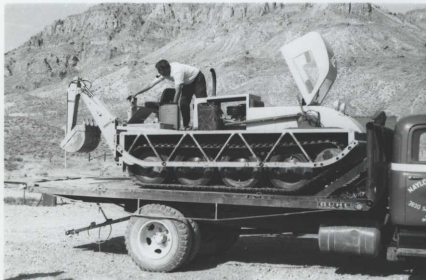
Refuge Bombardier tractor being returned from Naylor Equipment Co. in Salt Lake City where the backhoe was adapted and mounted. Depth of cut is between 6' and 7' and the present bucket is 18" wide. This attachment has increased the versatility of the tractor 100 per cent.
