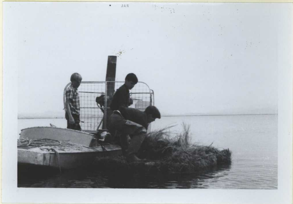
Dugway Boy Scouts earned credit toward merit badges while helping construct artificial islands. Below: Perforated steel planking shaped into "L's" and fastened together to form the frame for the islands. This frame is filled with baled hay and sodded with salt grass.
