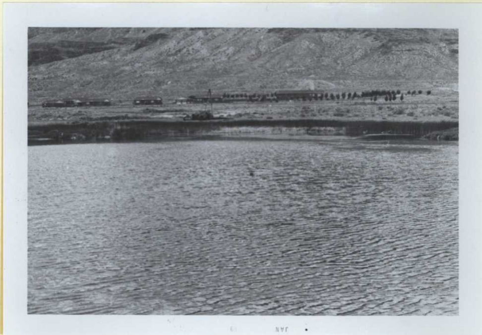
Above: Middle spring before removing the head. Below: After lowering the water level. Two second feet were gained by removing the pressure exerted on the spring by several feet of water.
