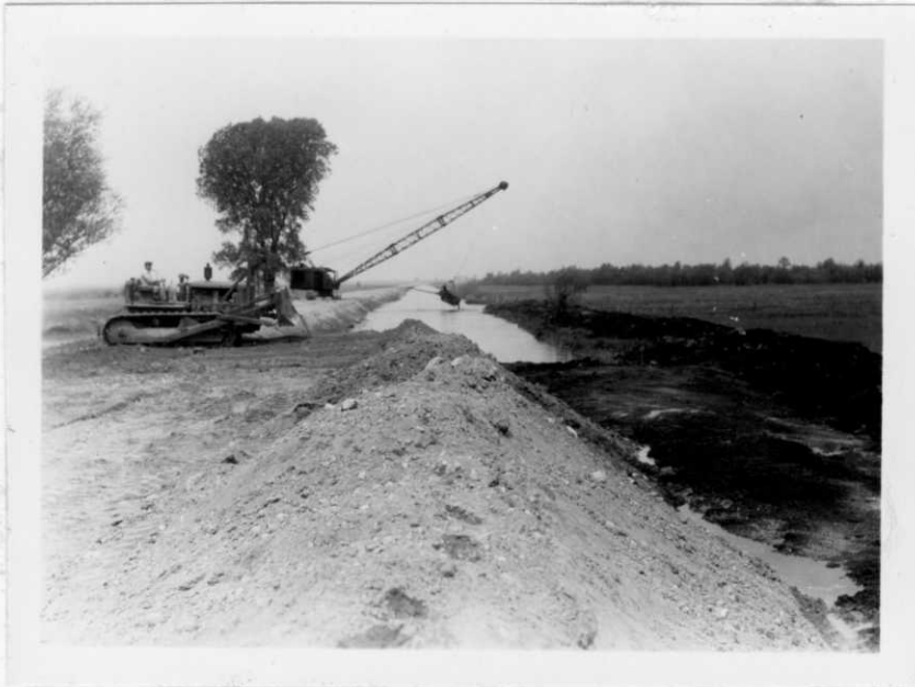
PUSHING DIKE FILL IN PLACE WITH BULLDOZER
