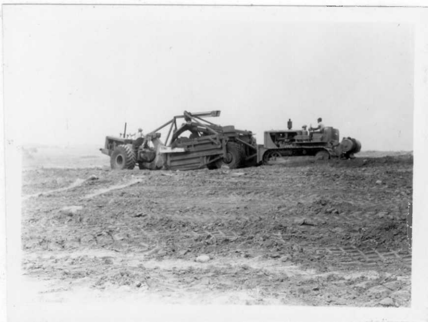
CLOSER VIEW OF PUSHER LOADING OPERATIONS.
