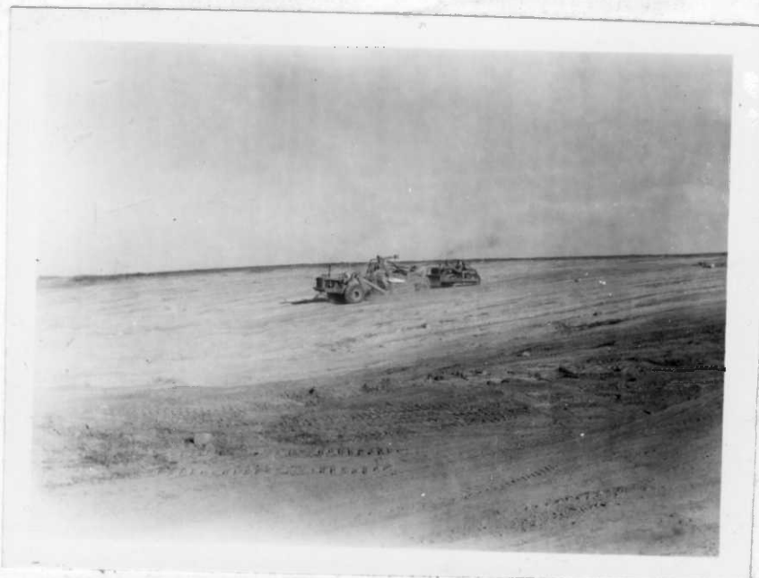
LOADING TOURNAPULL WITH AID OF PUSHER TRACTOR IN PIT ON OLD SCHREIBER FARM.
