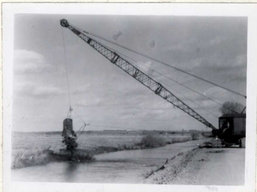
DRAGLINE EXCAVATING CORE TRENCH FOR DIKE IN WHEELER DITCH.
