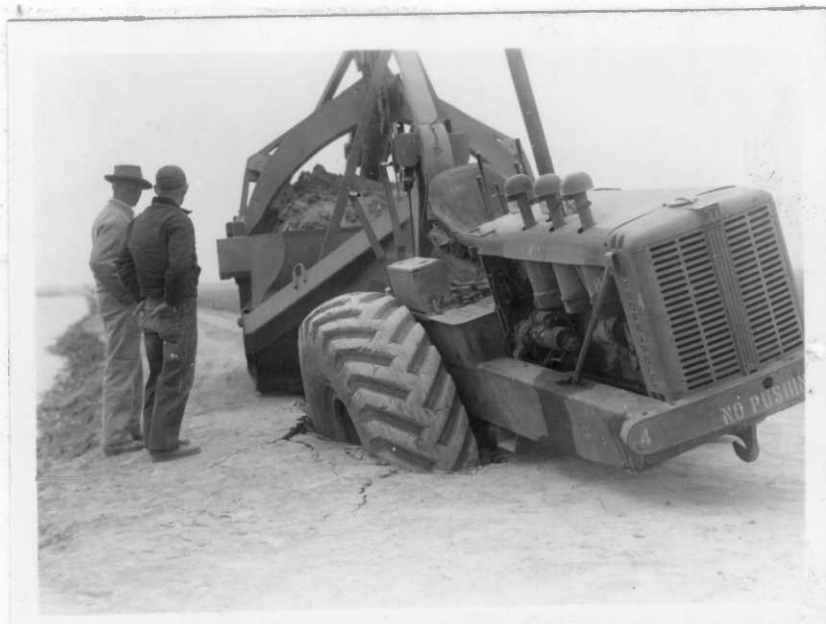
VIEW OF TOURNAPULL WHERE IT BROKE THROUGH THE HAUL ROAD ON FIRST TRIP OUT ON MAY 9, 1949
