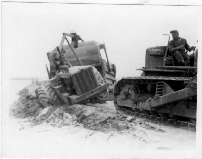
FIRST TOURNAPULL BROKE THROUGH HAUL ROAD AS IT PREPARED TO UNLOAD.
