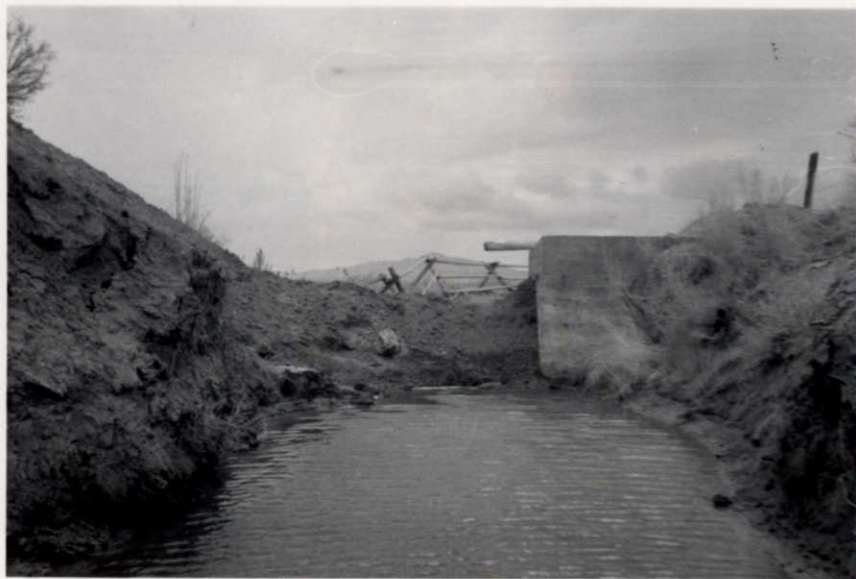
North slice of Hoge Dike after being dozed shut by our neighbors. This dam, about five feet in height, must be removed before the refuge can receive water. As soon as water conditions permit a new water control structure will be installed.
