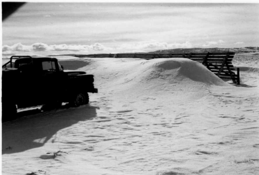
The State favors this portable-type structure but some picket-type fences are used effectively. Refuge fences are of picket type. R-9, #8
