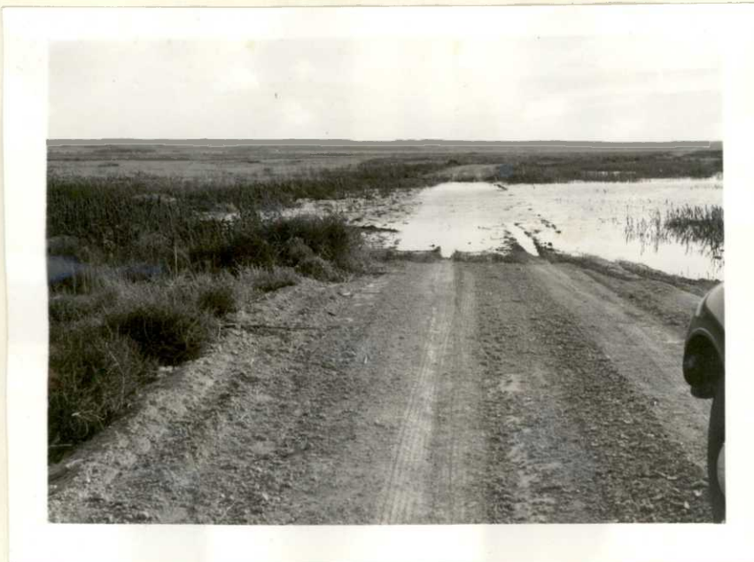
Water flowing over clay spillway in Dike 5.
