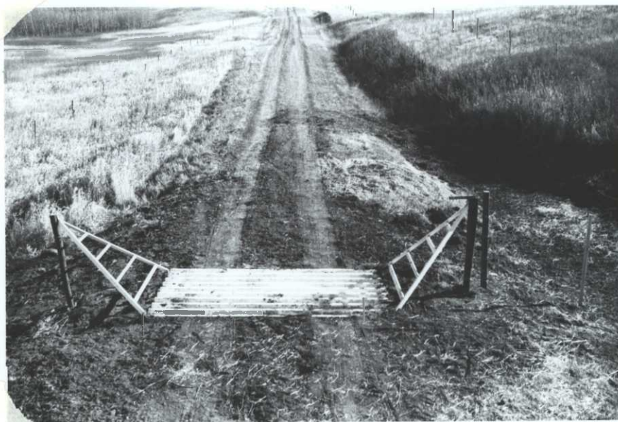
Plate # 4 Installation of cattle guard completed on Tower Trail
