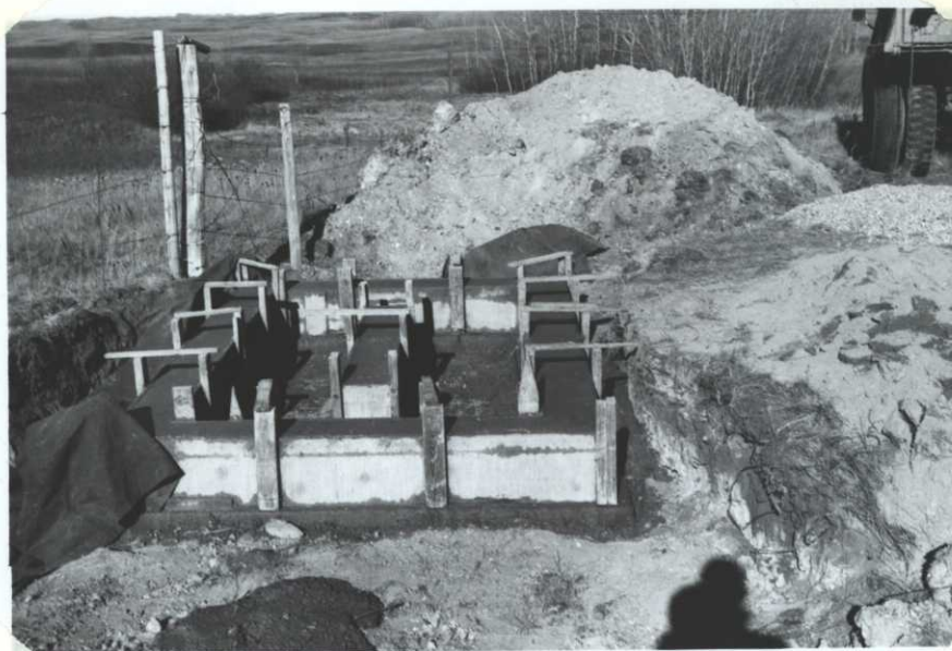
Plate # 3 Two section concrete foundation for cattle guards
