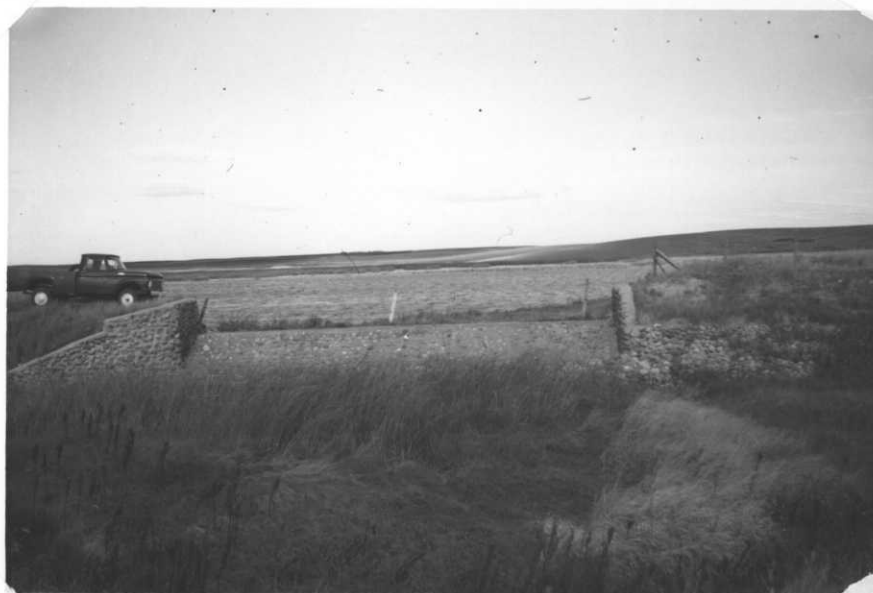
Combination rubble and concrete spillway at McLean Refuge should be replaced with reinforced concrete structure in near future.
