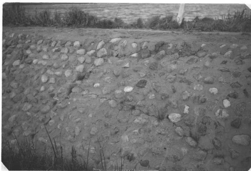
Close-up of rubble masonry spillway showing large cracks.
