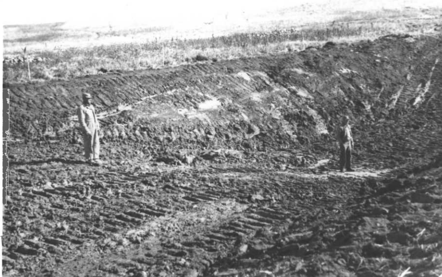
Stock watering dugout constructed to alleviate poor distribution of grazing pressure. Man on left is standing on the crest between the 4:1 and 7:1 end slope.
