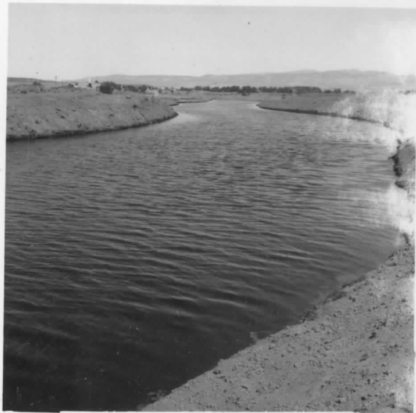
Pit River channel after flood control work. Banks planted to Refuge specifications of Intermediate wheatgrass, Ranger alfalfa, and others. (Larochelle)
