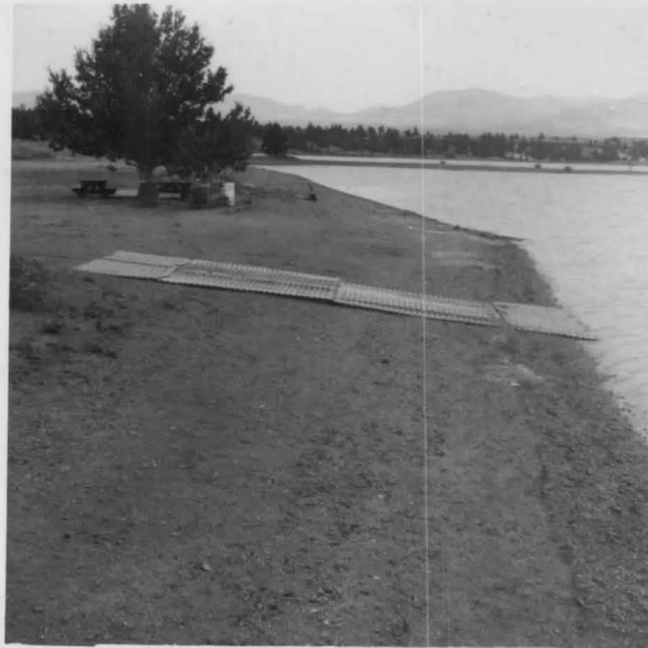
Aircraft landing mat material was used on Dorris Reservoir for temporary boat launching sites. (Larochelle)
