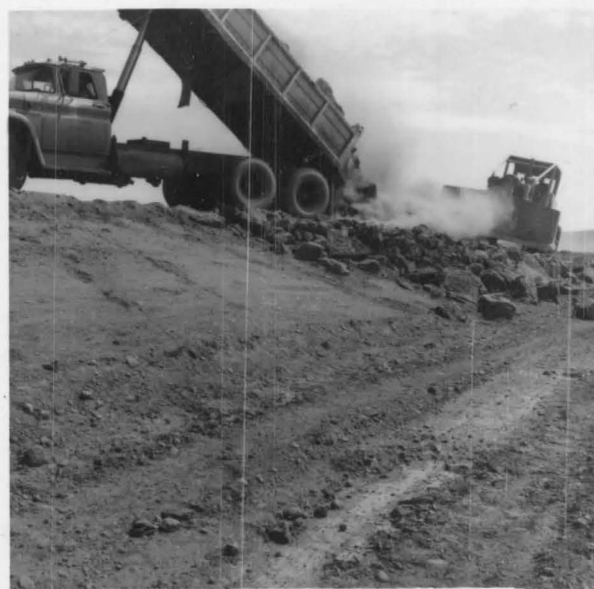
Flood damage of 1969 & 1970 to the North Grainfield dike was repaired by contract. 2,500 cu. yds. of riprap was placed to protect the dike from future floods. (Larochelle)
