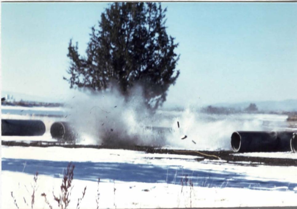
California Department of Fish and Game using prima cord to cut concrete pipes for use as spawning structures. MDC 2367, 11/30/88, BMS
