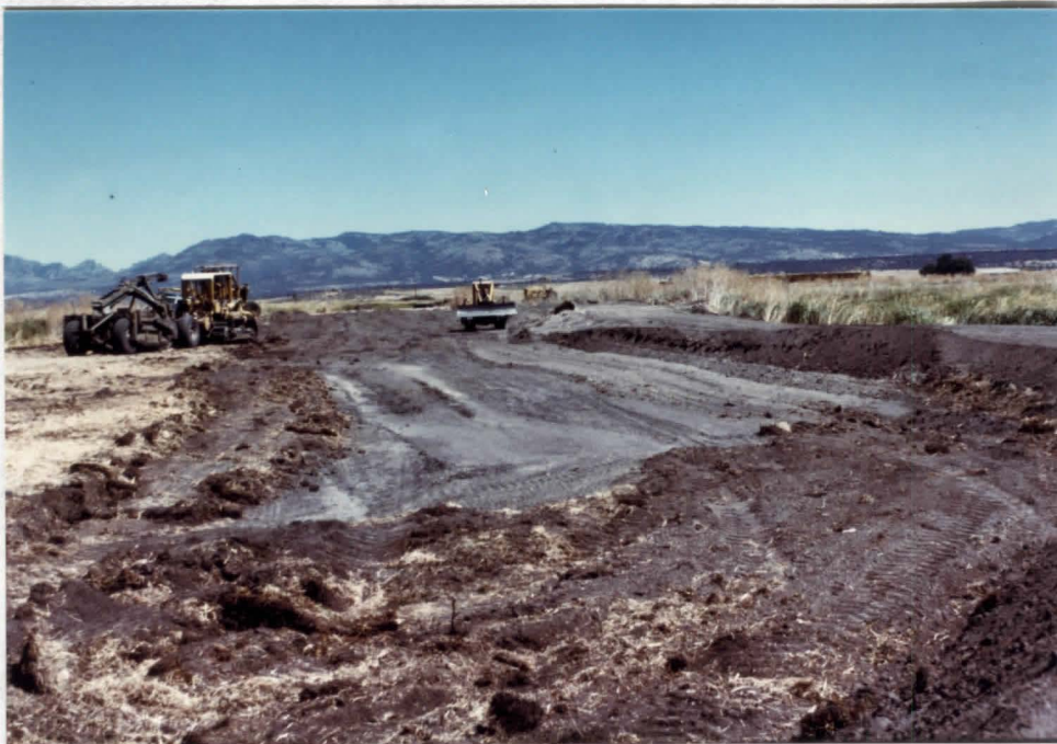
Cat and can being utilized in new pond construction. MDC 2353 8/23/88 TJM.
