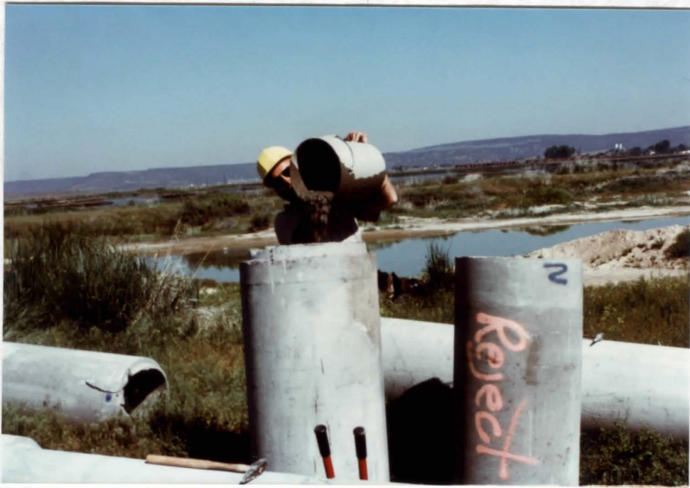
Maintenance Worker Storm pouring concrete into cut pipe for end wall. MDC 2424, 6/7/89 ECB
