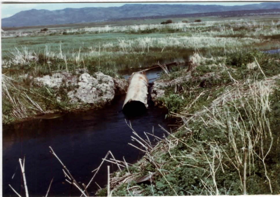
Water control structure on Pine Creek overflow which washed out in the preceeding winter. MDC 2416 05/22/89 ECB
