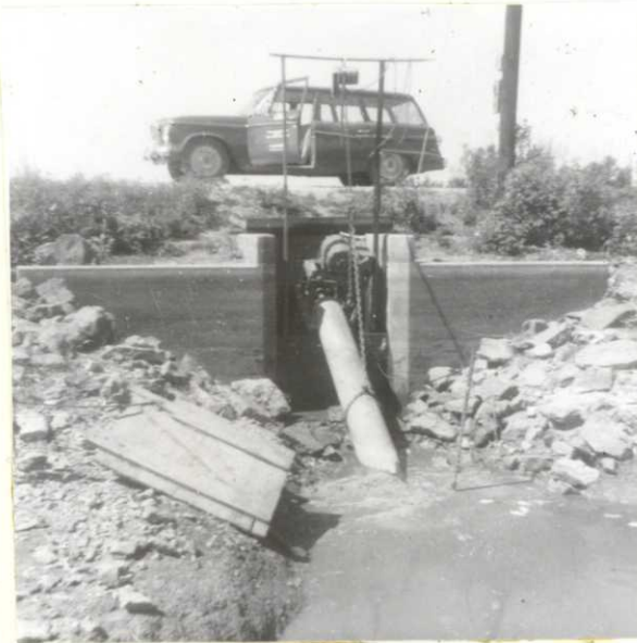
"The Cause of it All", twelve inch pump installed in the Fox Pond outlet structure.
