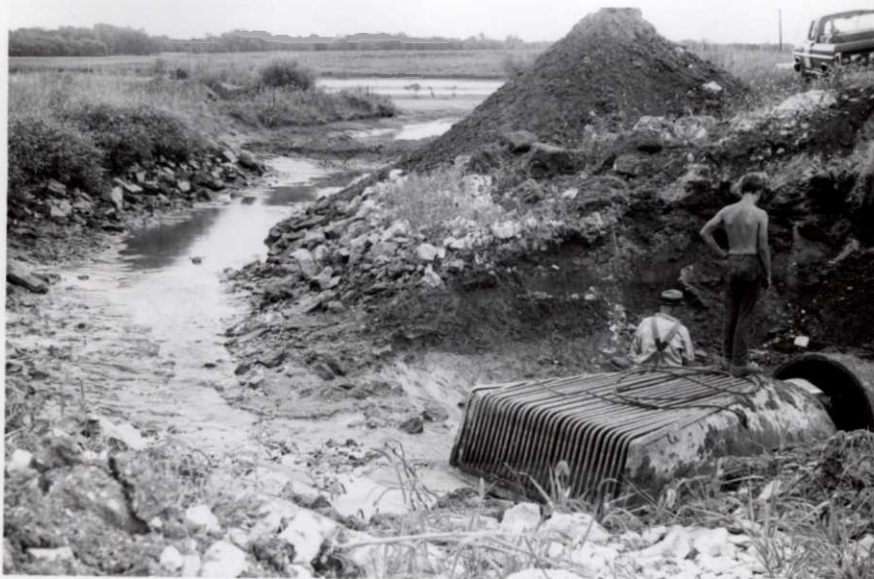
After 2 1/2 days of pumping, the concrete sections of the intake pipe came apart. Repairs made the pump inoperable for the rest of the year. Other "good news" was that the inlet ditch (shown extending into Fox Pond) was designed too small and will have to be doubled in width and rip-rapped again. This time by refuge personnel.
