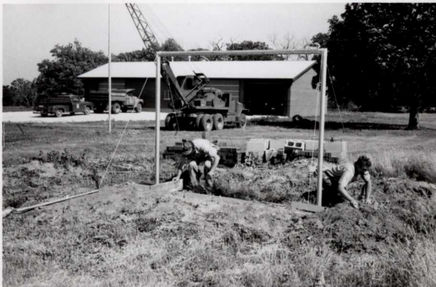
McNeil (left) and Manager Weier (right) are shown at work on the foundation for the Louisa headquarters sign. In the background, an aluminum flagpole is held in place by the refuge motor crane until the concrete in the base sets. R202, P-1 EMW June 1968
