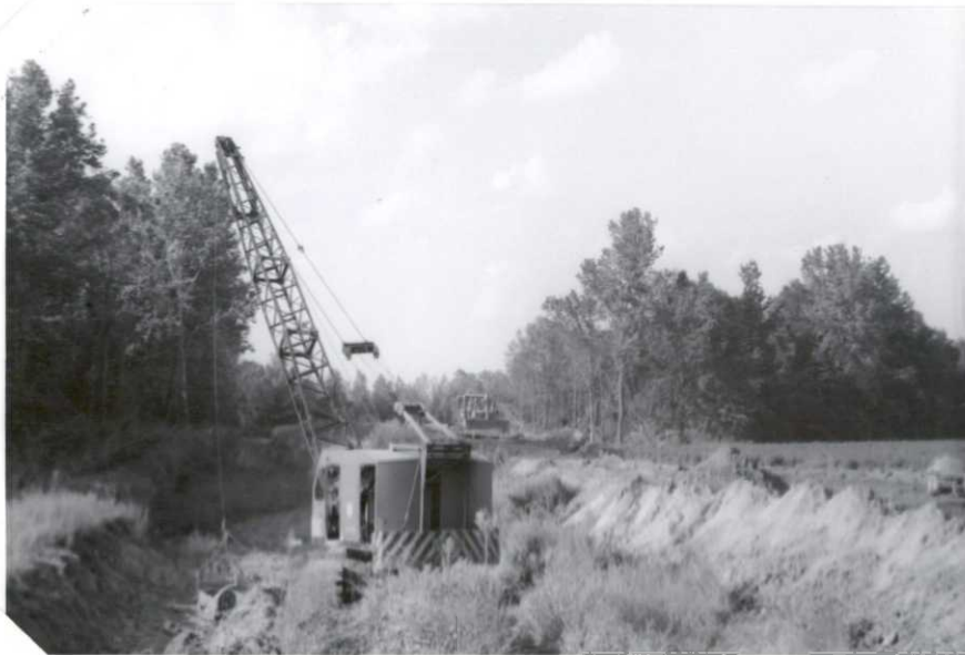
Completing the fill on the Burris Road with the dragline and Bulldozer.
