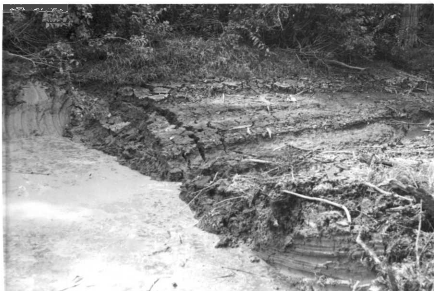
Figure 11. Ditch #5, the main drainage ditch for Monopoly Marsh, had not been cleaned since being constructed in 1915 and had completely silted full.
