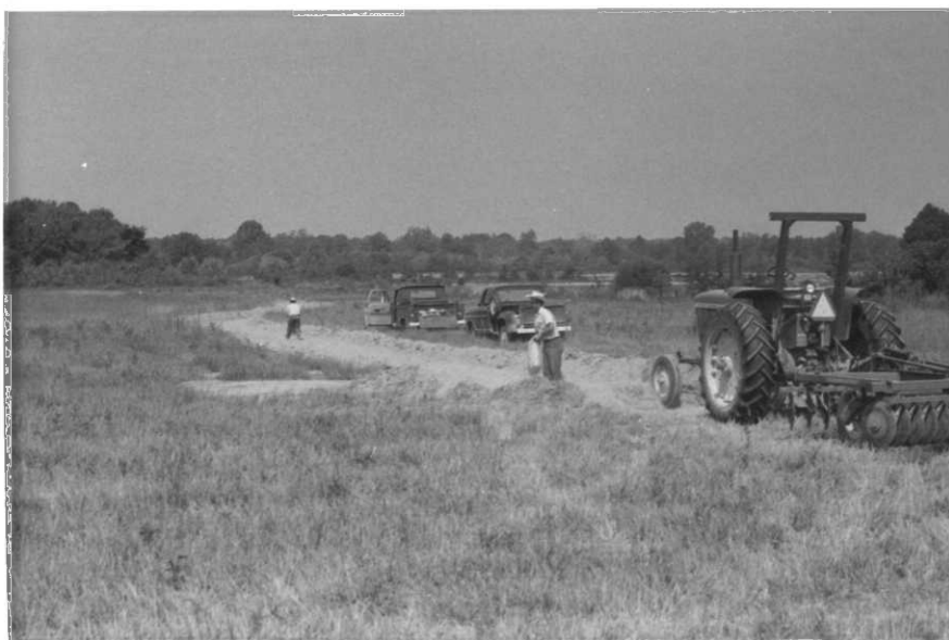
Figure 9. Spring rainfall caused severe erosion on a newly seeded pasture at Flatbanks. This 12 foot waterway eliminated the problem.
