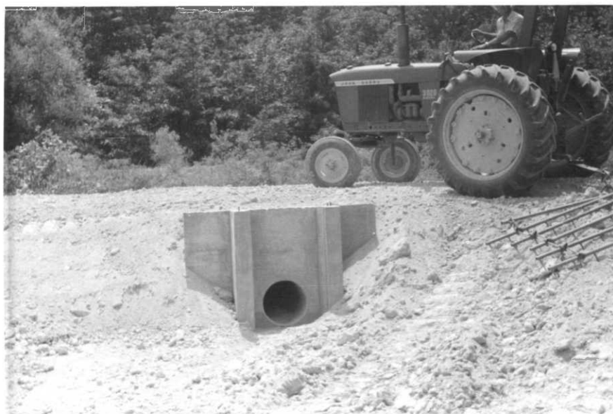
Figure 8. Levees were pushed-up and seeded, and stop-log structures were constructed on most of our moist soil plant units.
