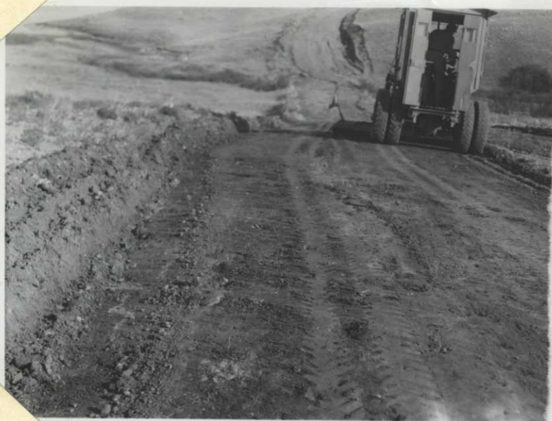
Blading patrol trail on the South side of the Lake. No. 557 10-26-50
