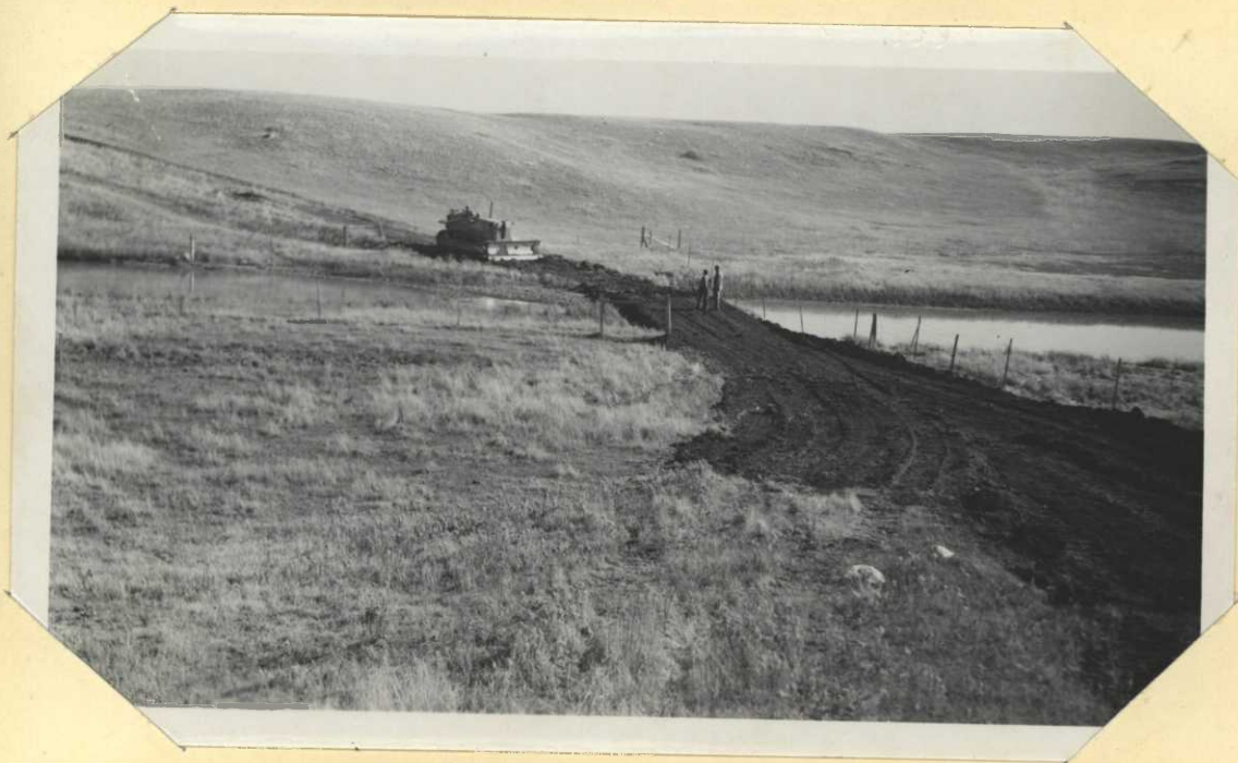
Filling in washout in patrol trail.
