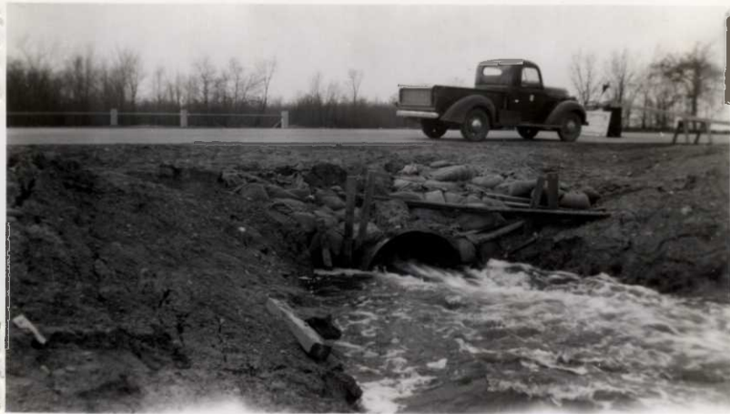
Incomplete Connecting Spillway - March, 1942
