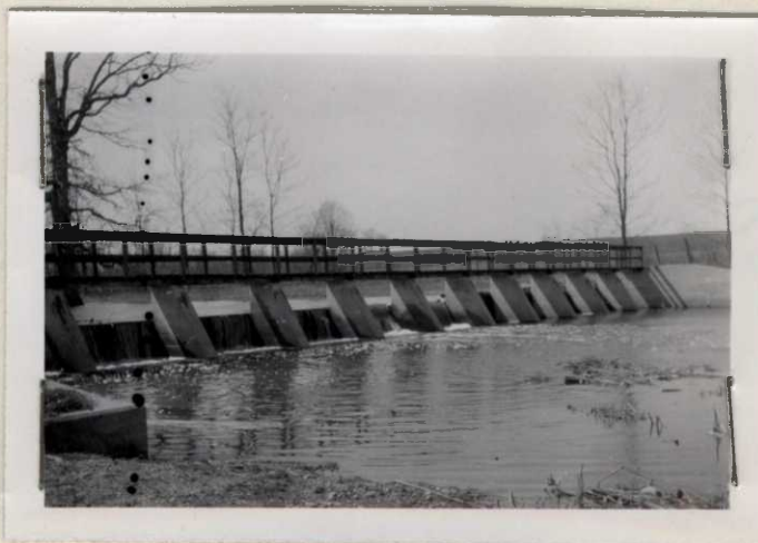
Storage Pool Spillway With Level Just Above Pool
