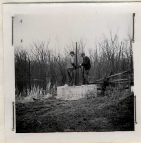
Greasing Controls on Black Brook Spillway Gate
