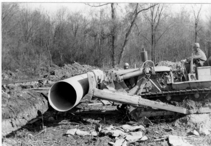
Culvert pipe carried to site with the D-6
