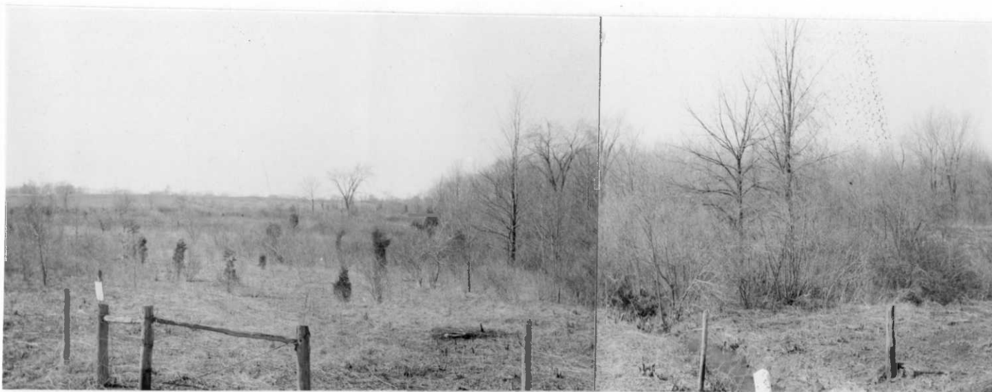
- View, BEFORE, of clearing carried out for construction of the east end of dike for development of our long-proposed Big Spring Pool. Rotary brush cutter cut all but the heaviest material. Ditch cleared out to point of outlet of new control structure.
