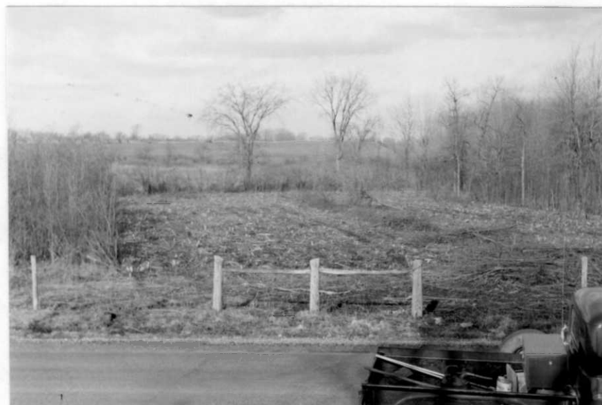
- Note brush piles in center left from the initial 8 foot swath cut by hand. Nothing left to burn following the rotary brush cutter.
