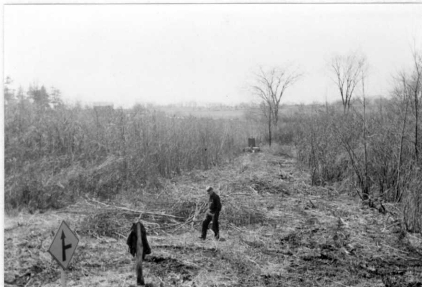
- A path was cut out by hand tools so that Model 25 International brush cutter could get started in this alder. Machine handled alder up to 3-1/2 inches through by taking a narrow swath at a time. View is along path of dike to be constructed to enclose 150 acres Big Spring Pool.
