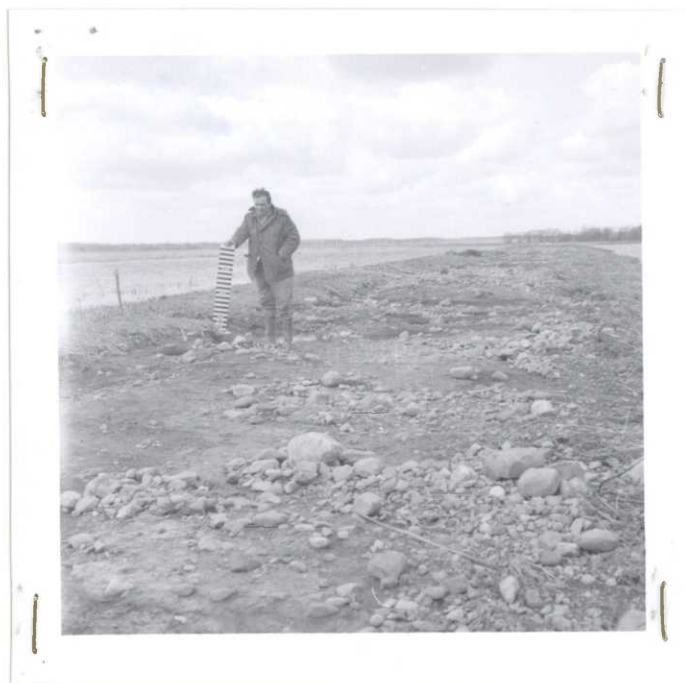
Severe water damage to Main Pool dike. Note how well sod areas held up-compared to gravel roadbed.
