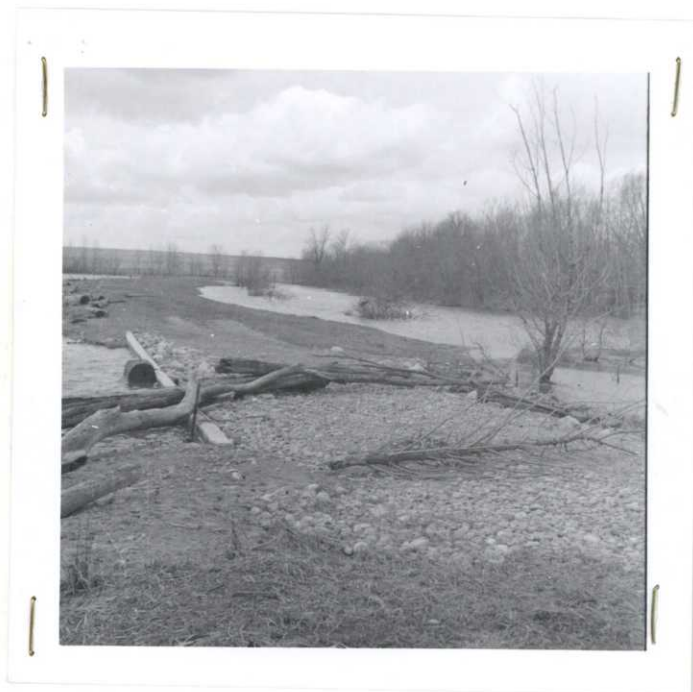
Debris left by high waters on equalizer of Storage Pool. Retainer wall helped hold stone in road area very well. Little or no wash-out of stone was noted.
