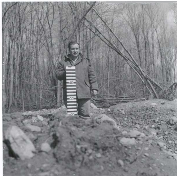
Washout of new Spring Pool dike adjacent to Route 89, south of Thruway.
