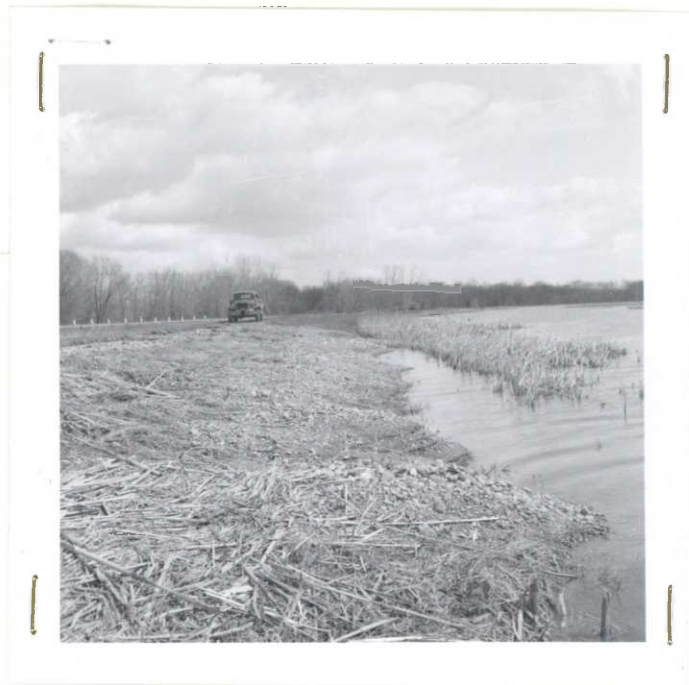
Inside of Main Pool dike where flood waters deposited gravel from road bed area on dike.
