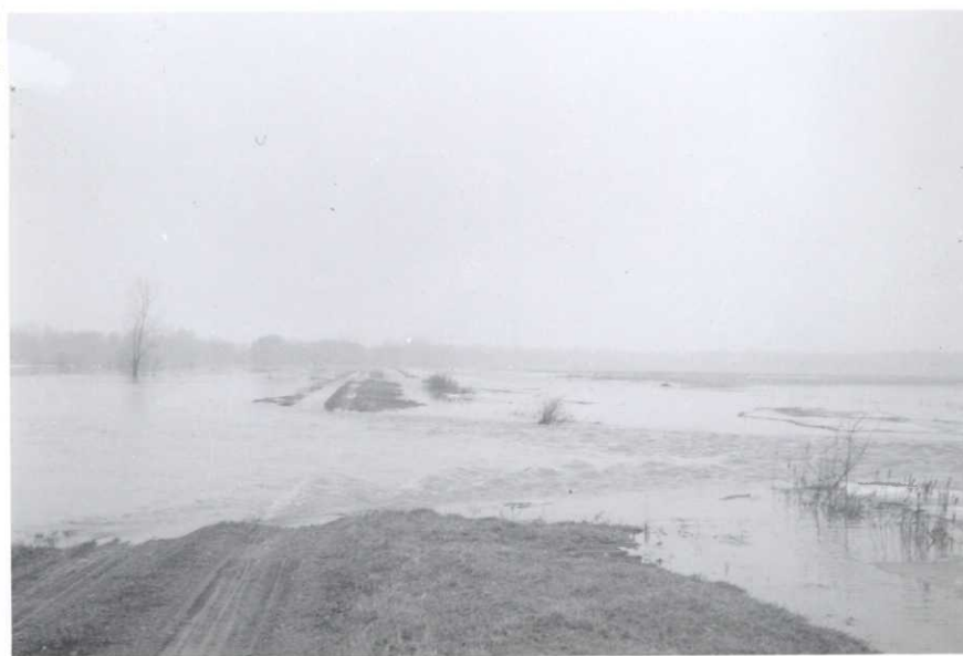
Main Pool equalizer filled with flood waters. Water is about 4' deep in center and about 100' across on top.
