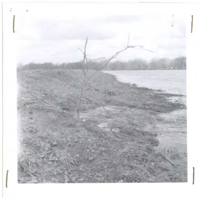
Results of our dikes worst enemies. Muskrat burrowed from inside dike and woodchuck burrowed from outside (view) thus weakening dike and allowing water to cut through.
