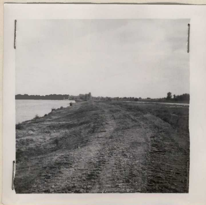
Dike Finally Roughed Into Shape
