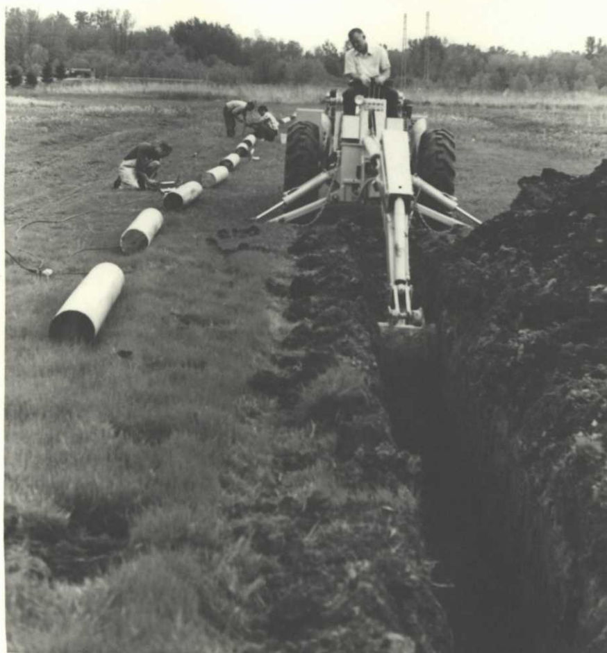
A new pipeline rectifier was installed under permit by Mobil in Field No. 8 near headquarters. It was buried deep enough so as not to be a hazard to our agricultural activities.
