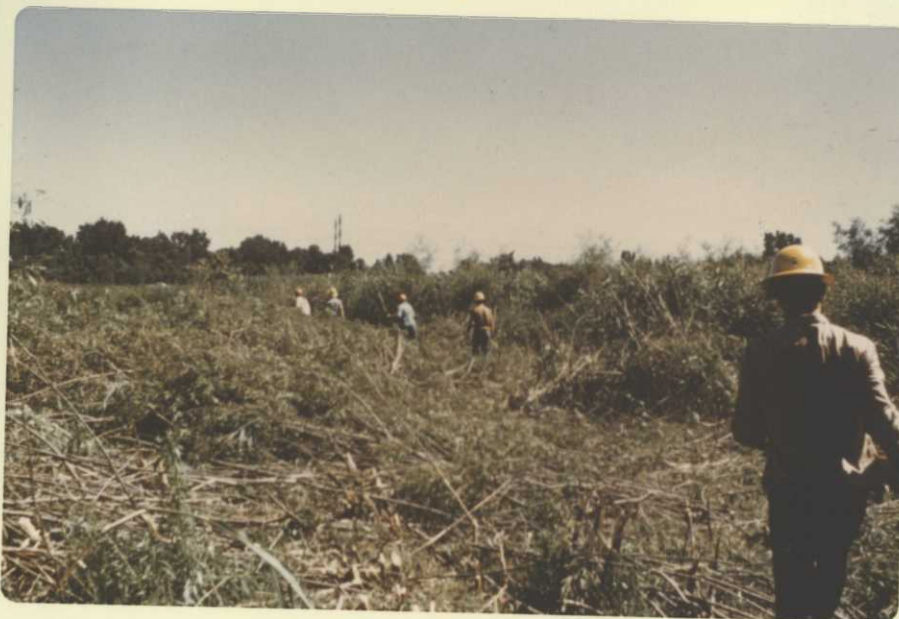
Enrollees used axes, brush hooks, mattocks, and crosscut saws. Boots with hard soles and box toes, hardhats, and gloves were required for most work projects. There were no reportable accidents during the 8-week period (Amen!)
