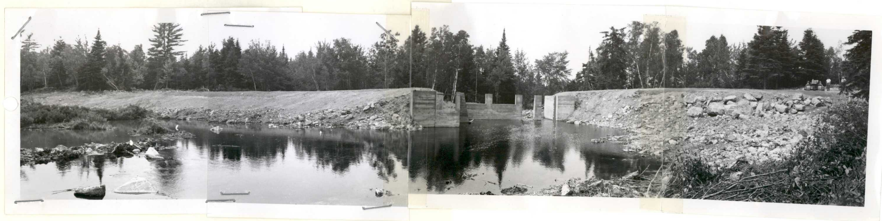
Howard Mill Dam - Top: - Looking upstream at earthen dam and cement spillway and fishway at completion of cement work. Prior to seeding etc.
