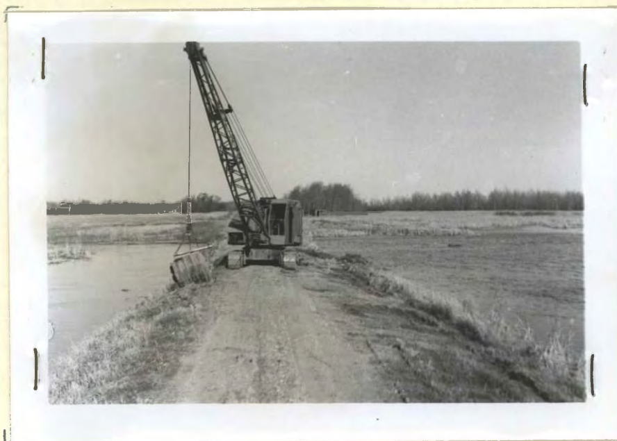
6. The dragline was put into use after ice broke up sufficiently to permit fill to be obtained.
