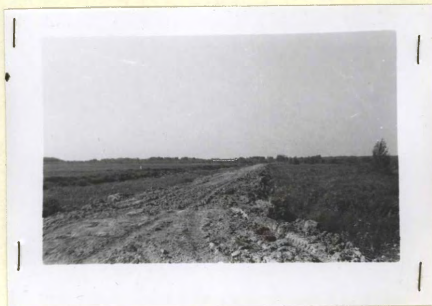
Section of newly completed "ring dike" before sloping and dressing - Madsen Pool.
