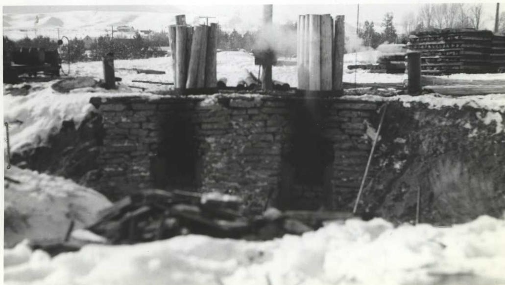
The creosote treating plant was much improved when moved to the wood yard. This shows the plant in operation.
