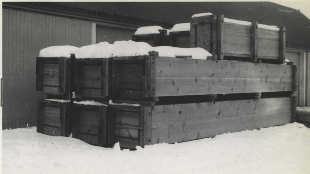
Large and small wooden water tanks, constructed under soil and moisture project, for installation at new springs.
