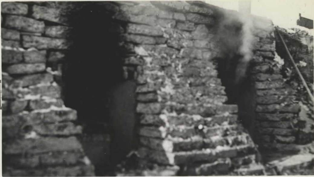
Two tanks were sunk at the edge of a gully bank, which was excavated. Banks were walled up with broken up concrete slabs, salvaged from the CCC Camp. Fire boxes are under the tanks.
