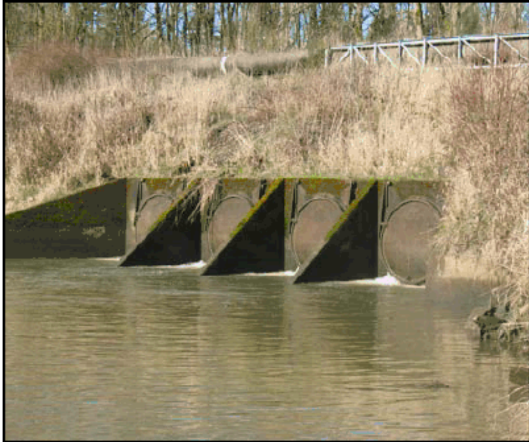
Figure 2. Top hinge cast iron tide gates on South Deer Island Slough, 2009.
