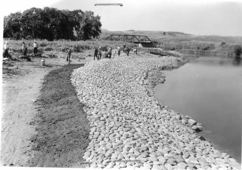
CCC crew relaying riprap on the down-stream side of Dam 320 R115-2, Sept. 1940
