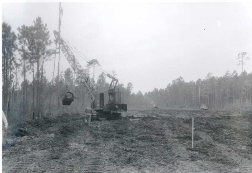
Removing peat from right of way for con- struction of sill.
