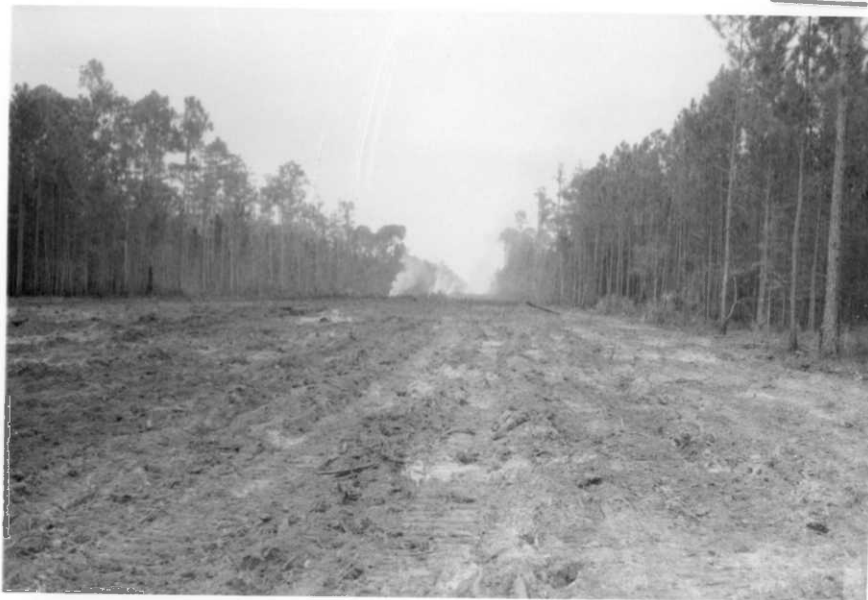
Sill right of way cleared and grubbed.
