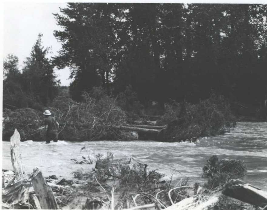
The channel was clogged with uprooted trees -- these had to be removed to avoid aggravated damages.
