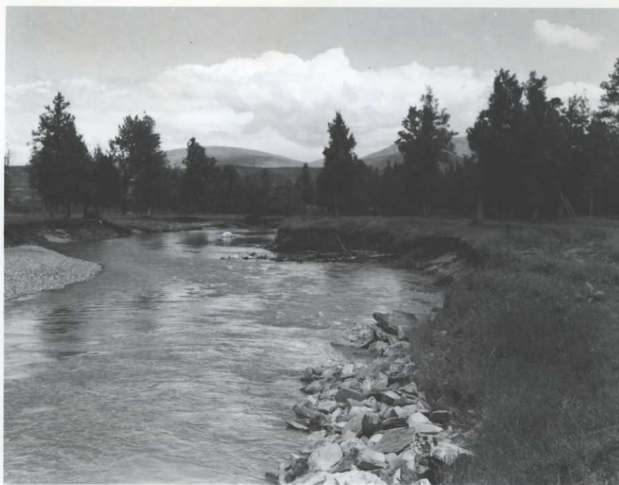
Bank erosion and rip-rap loss.
