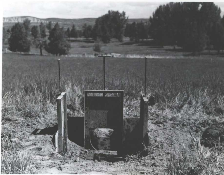
Newly installed three-way headgate in one of refuge hay meadows.
