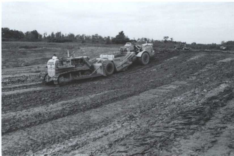
Contract dike rehabilitation equipment at work. No. 65-11-5A6 - Manke - 06-09-65
