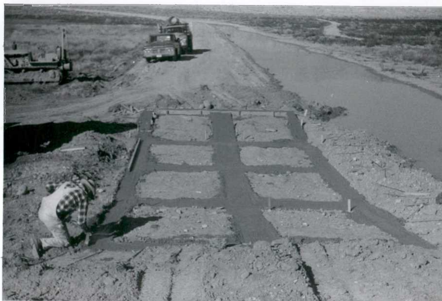
Pour the concrete and the foundation is set for the slab.
