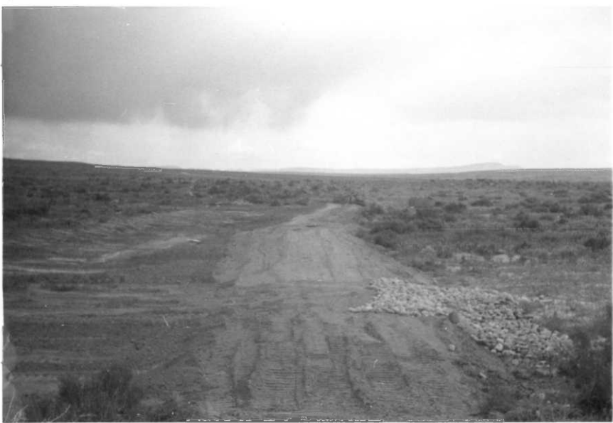
Same dike as seen looking across the top. Note rip-rap on down stream slope of spillway.
