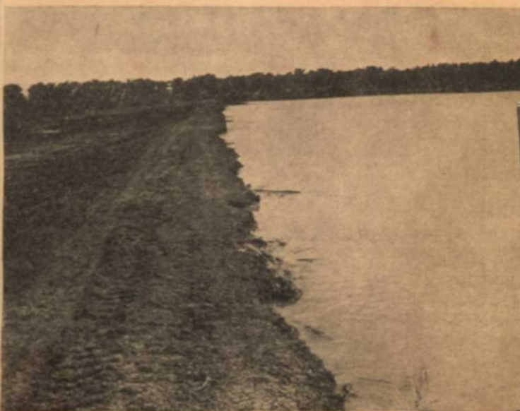
FLOOD WATERS threaten to delay construction last spring at Ouray National Wildlife Refuge. High water laps at a dike after it was raised two feet at Leota Bottom.
