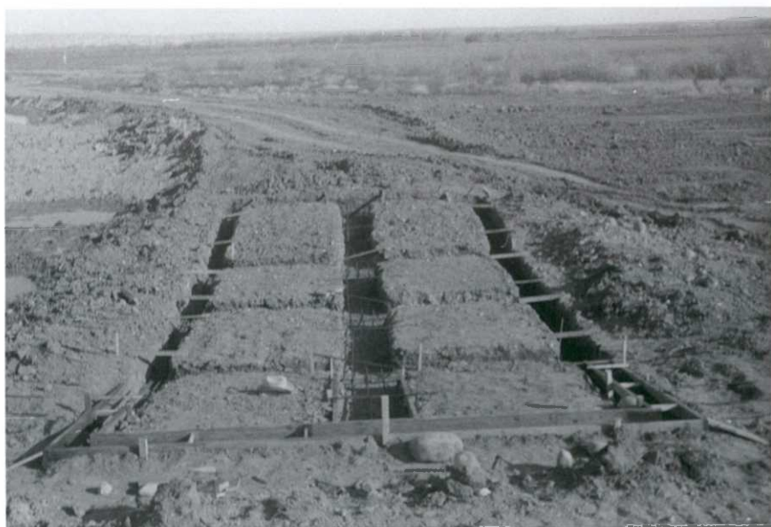
Open footings and a lot of reinforcing steel mark the beginning of a water gap constructed in the West Canal Protection Dike.
