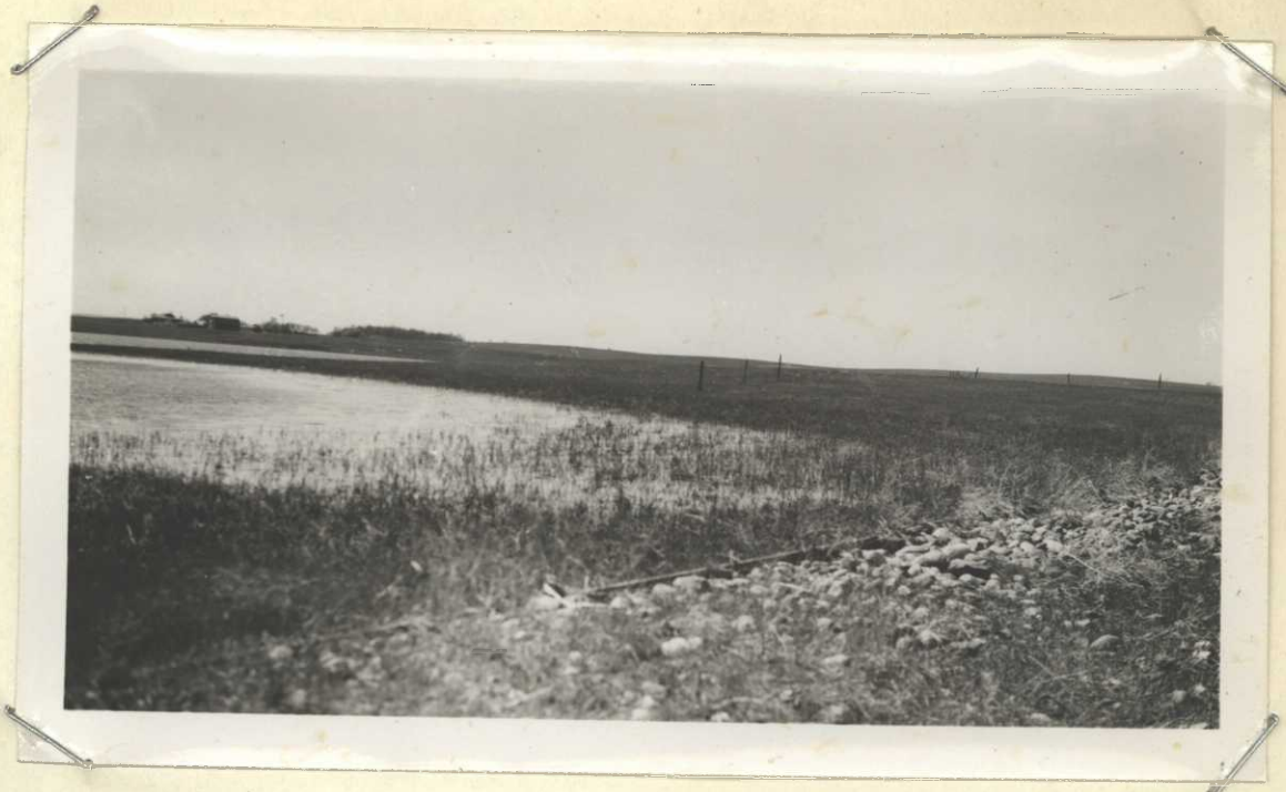
Bonehill Creek Refuge: 6-3-50 - Shows water level still near spillway level - water merely flows around the end of the dam through a natural well grassed draw. R100-1.
