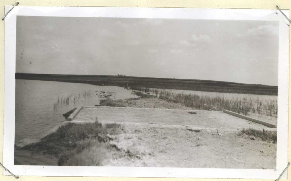
Stoney Slough Refuge; 8-8-50 - Shows the grade crossing on the refuge between units 4 and 5 after it was damaged by the spring run-off. R102-1.
