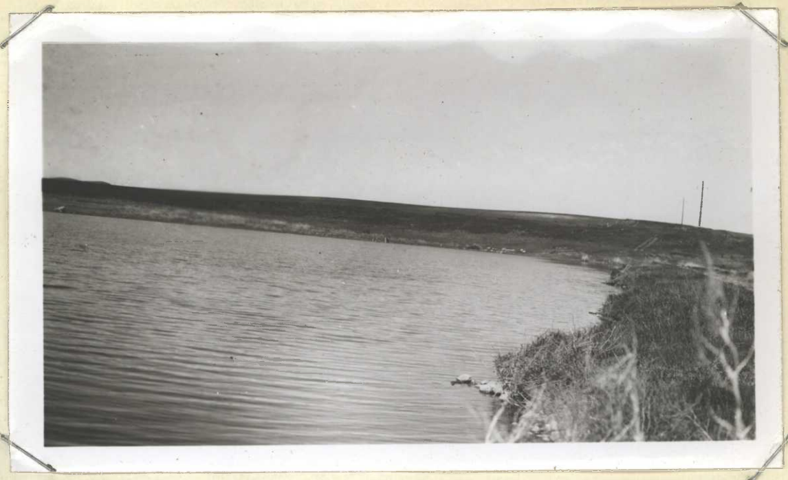
Hobart Lake Refuge: 6-3-50 - Shows some erosion on dike caused by wave action during high water. R100-3.
