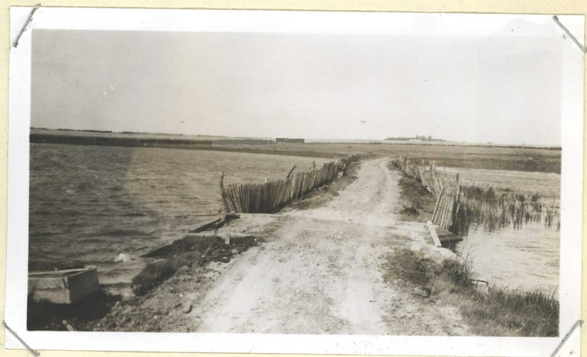
Stoney Slough Refuge: 8-17-50 - Raising of grade completed and gravelled. Shows old snow fence put in to prevent wave action on new grade. R102-3
