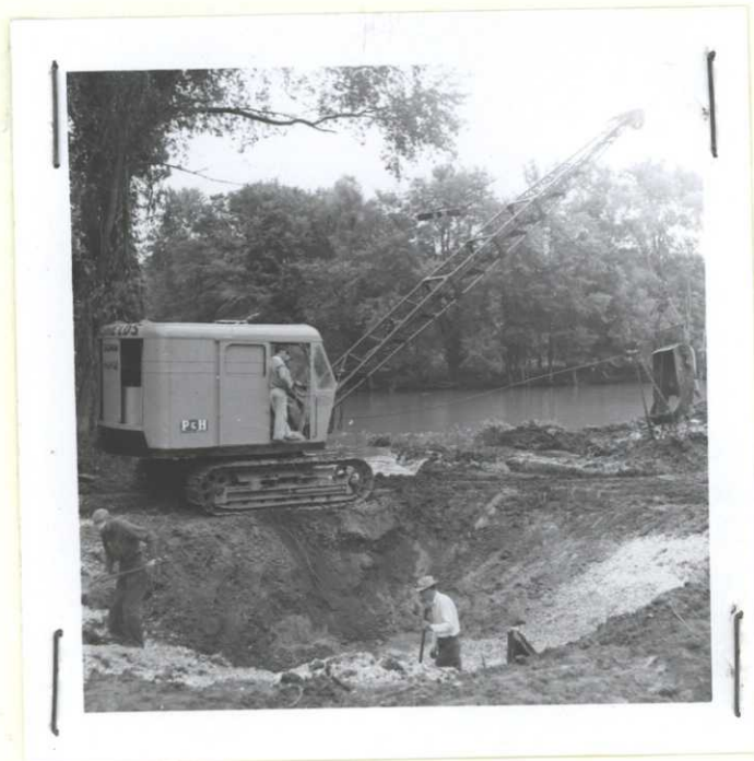
Installation of 48" diameter discharge pipe with flap gate on Watson Tract to provide new outlet into the Cass River for water collecting on farm land within protective dikes.
