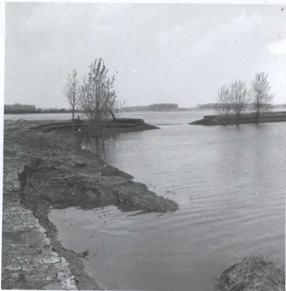
Break in riverside dike and example of erosion on slopes.
