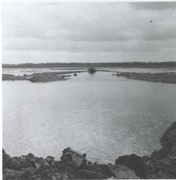
Washout and debris in field in front of an area where water broke through dike.
