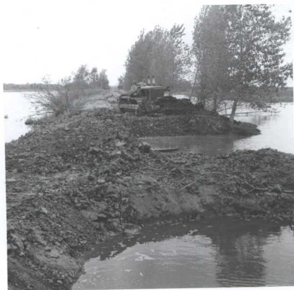
There is little material within reach for fill when breaks occur. Breaks closed temporarily with bulldozer and later built up by dragline.
